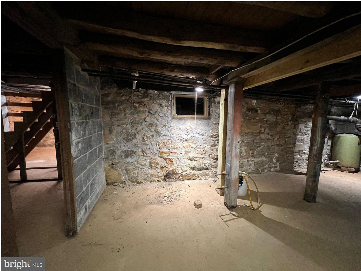
Figure 9: Interior photo of the basement showing stone foundation.
