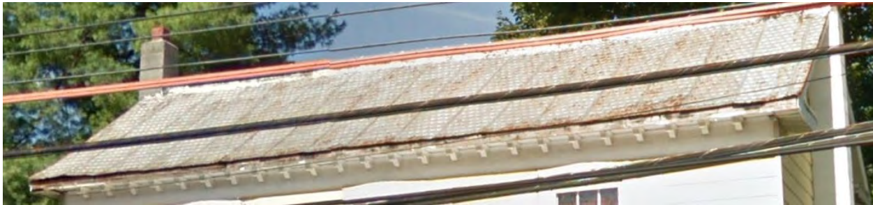
Figure 22: Google Streetview image of the roofing showing the 17 existing panels, shingle texture, and deterioration.
