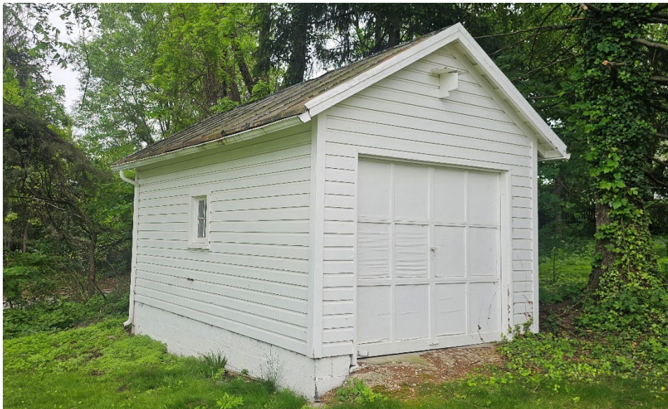
Figure 15: View of the one-car garage in the rear yard of the property, 2025.
