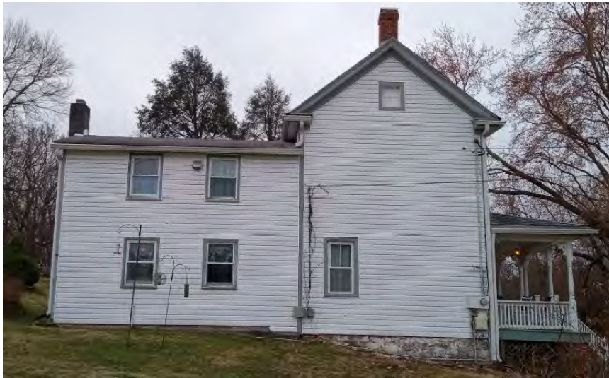
Figure 10: Existing left-side (northeast) elevation photograph showing the aligned fenestration and existing two-over-two window on the main block.
