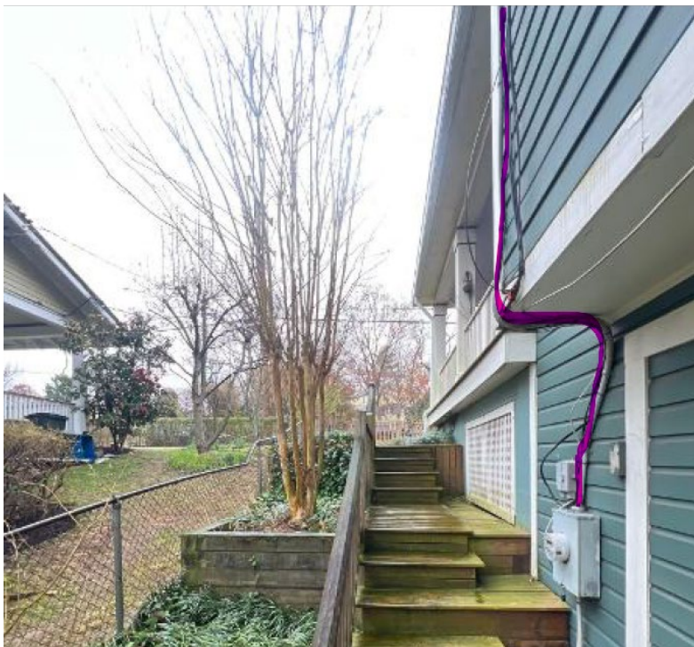
Utility Meter after Install
