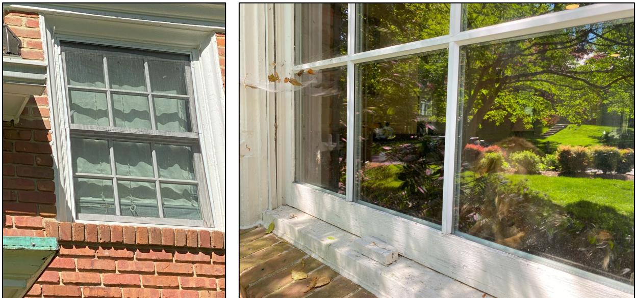
Figure 5: Wood windows on the second story (left, 2025), and detail of wood windows on the second story with clad grilles (right, 2025).
