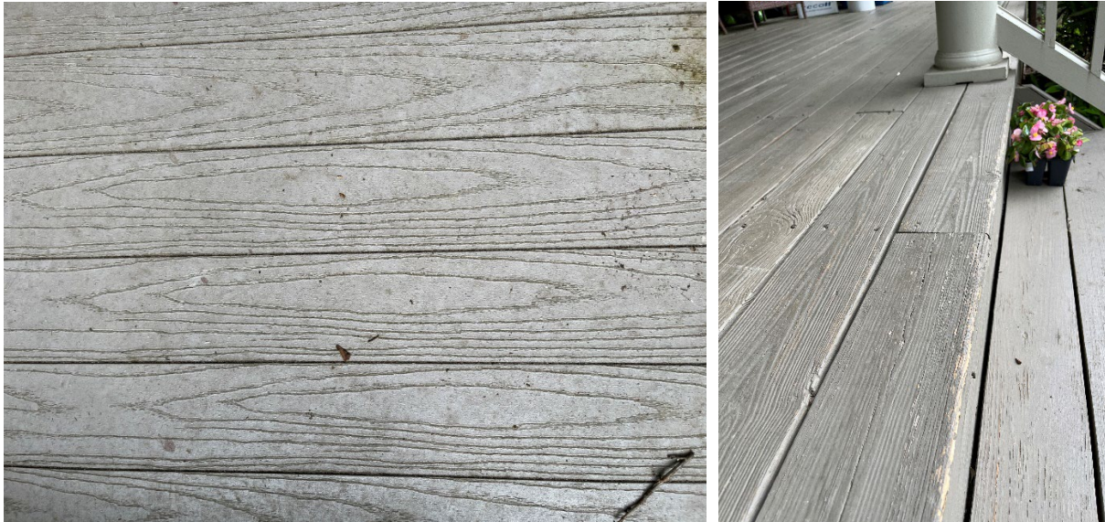
Figure 6: Exaggerated wood grain texture of installed Timbertech flooring (left) does not replicate actual wood texture (example of wood texture on the right)
