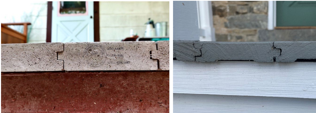
Figure 7: Installed boards on the subject property (left) and wood boards (right). The tongue and groove joinery appears to have a manufactured, rather than milled, appearance. Additionally, the edges do not replicate the appearance of actual wood grain.
