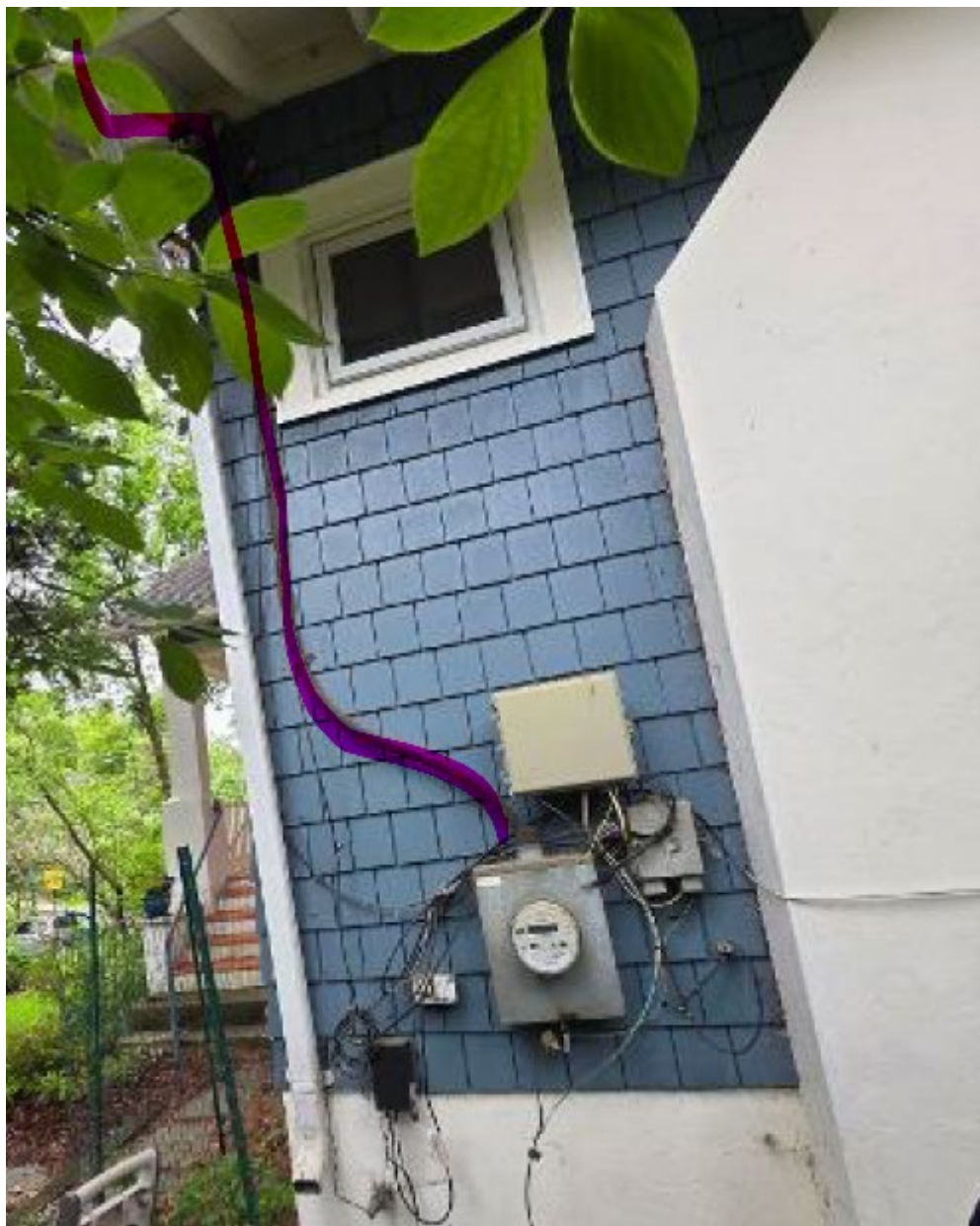
Utility Meter after Install
