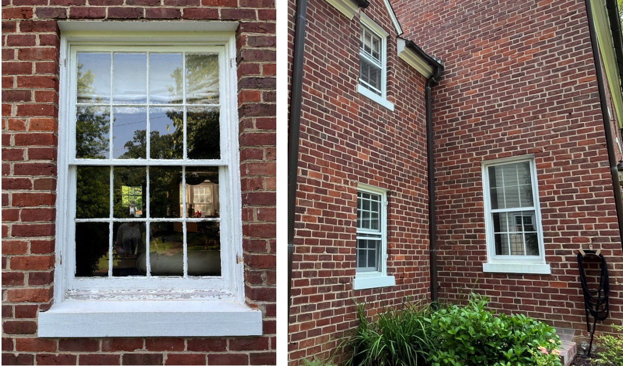
Figure 3: Photo of existing 8/8 double hung sash windows (left) and 6/6 double hung sash windows (right).
