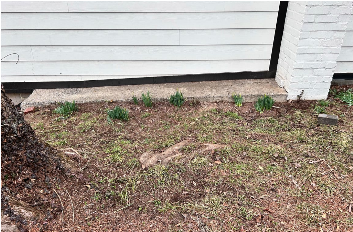
Figure 12: Proximity of roots to foundation, including some cracking along supplemental foundation wall, 2025 (Historic Preservation Office).
