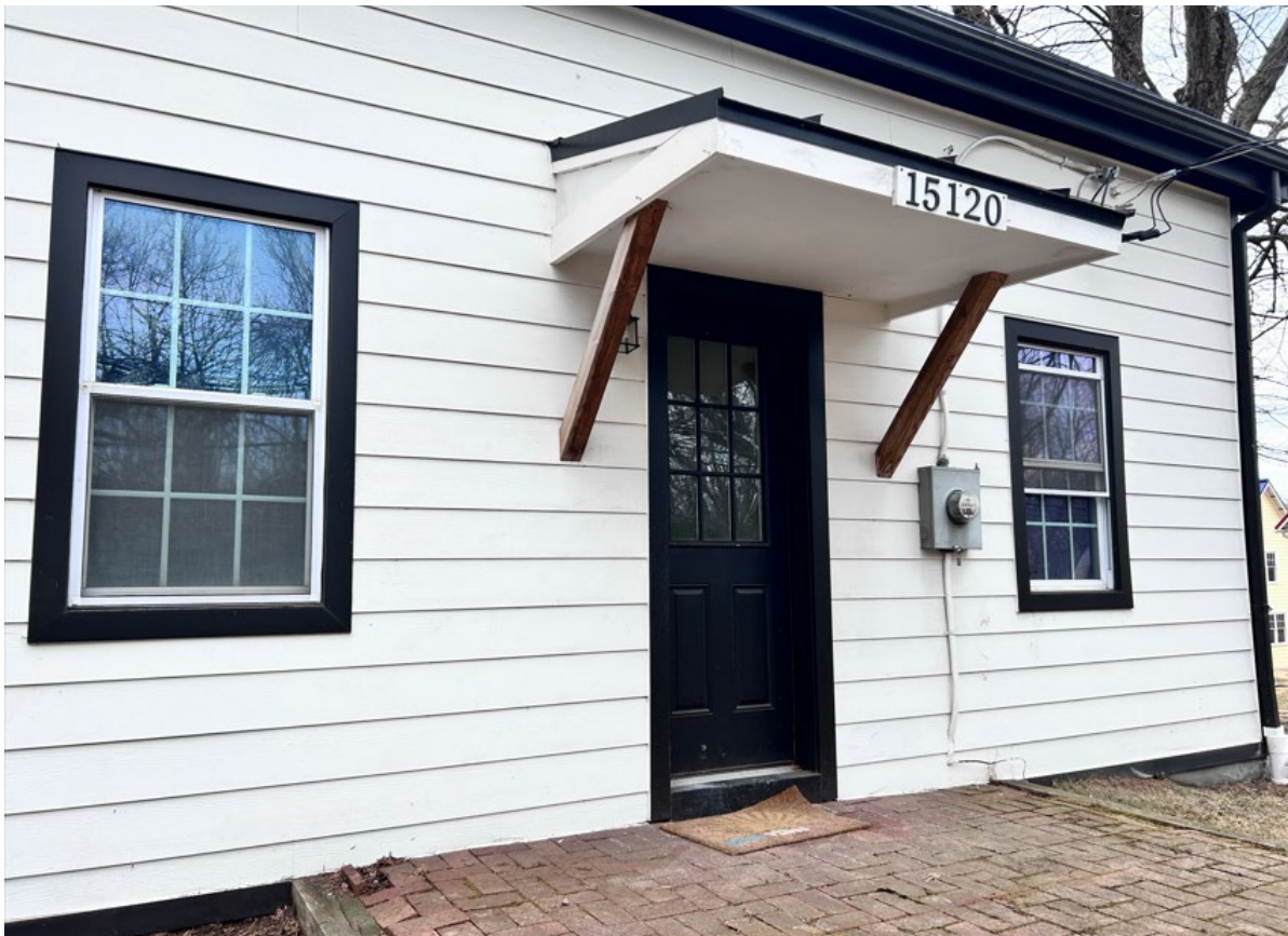
Figure 16: Detail of the front façade of the subject property with replacement siding, February 2025 (Historic Preservation Office).
