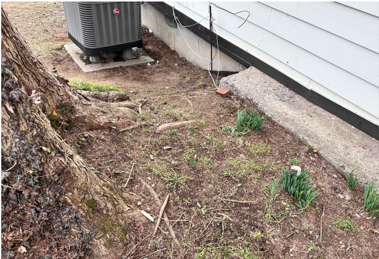
Figure 11: View of the proximity of the tree roots to the building foundation, 2025 (Historic Preservation Office).
