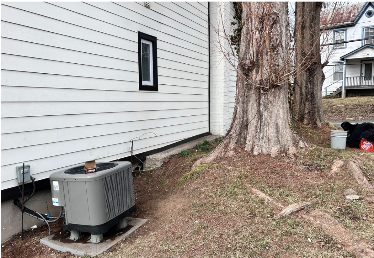
Figure 13: View towards Barnesville Road showing the proximity of the tree roots to the building foundation, 2025 (Historic Preservation Office).
