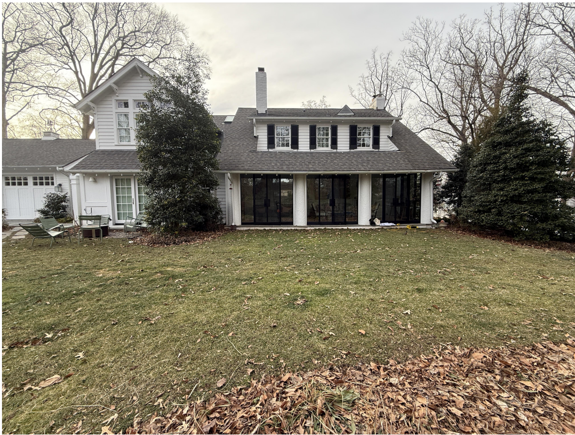
Photo 1: Existing East side of the house- Showing porch doors to be removed and second floor bedroom to be renovated
