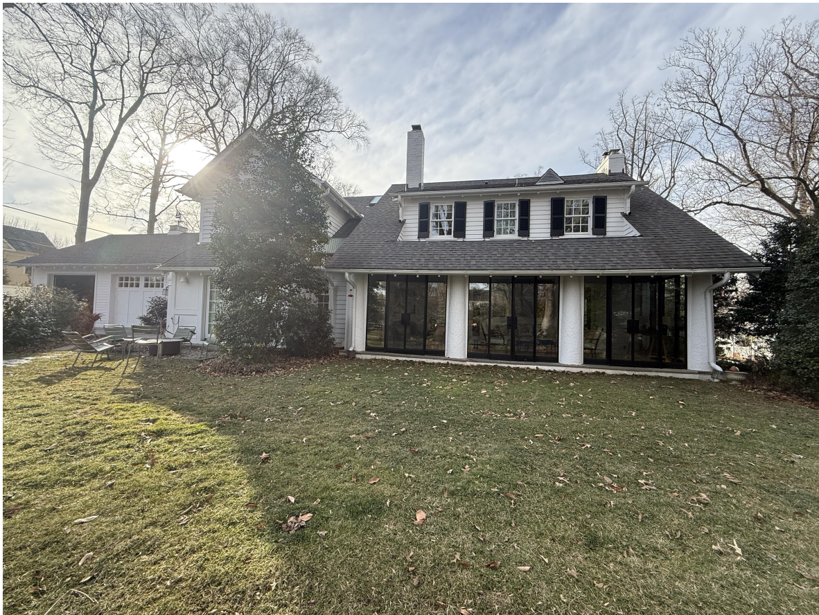
Photo 3: Showing East side of the house- Porch doors to be removed
