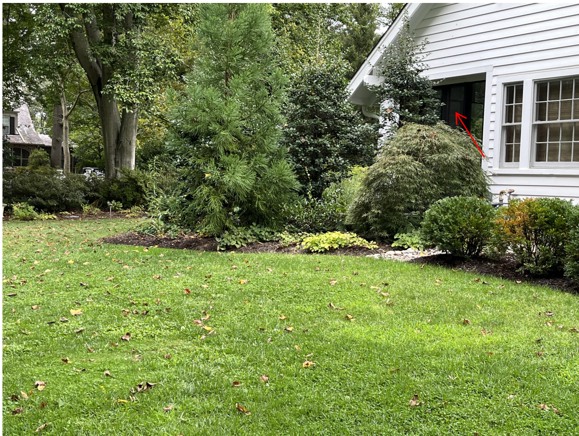
Photo 2: North-West corner of the house. Showing porch window to be removed
