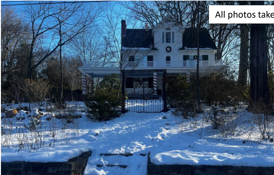
Front of house with street in foreground
