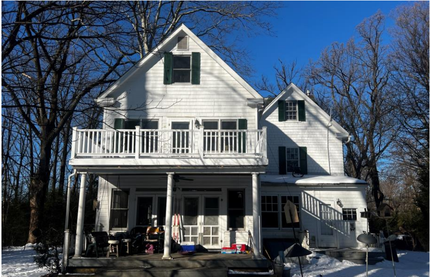
Rear of house
