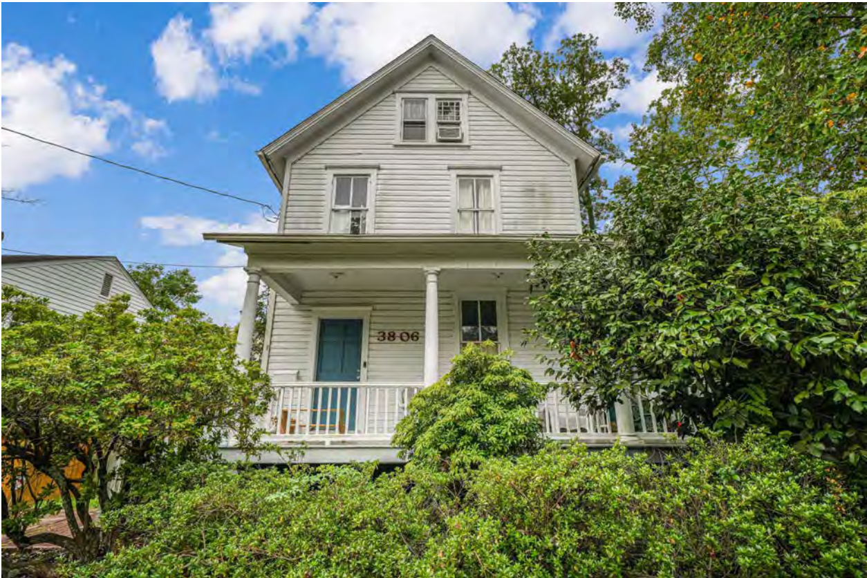
3806 Williams Lane - North façade (facing Williams Lane)
