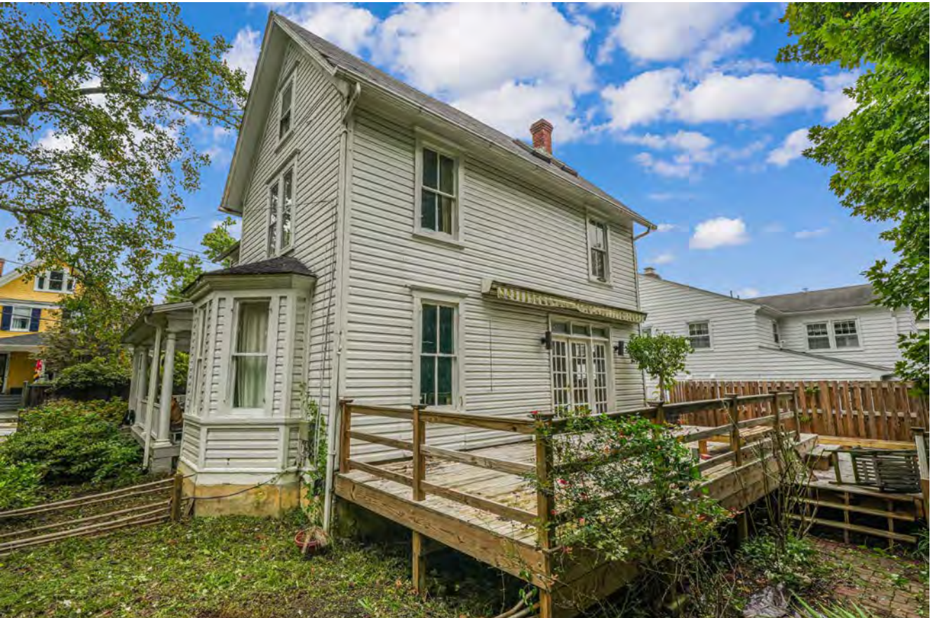
3806 Williams Lane – Southwest corner
