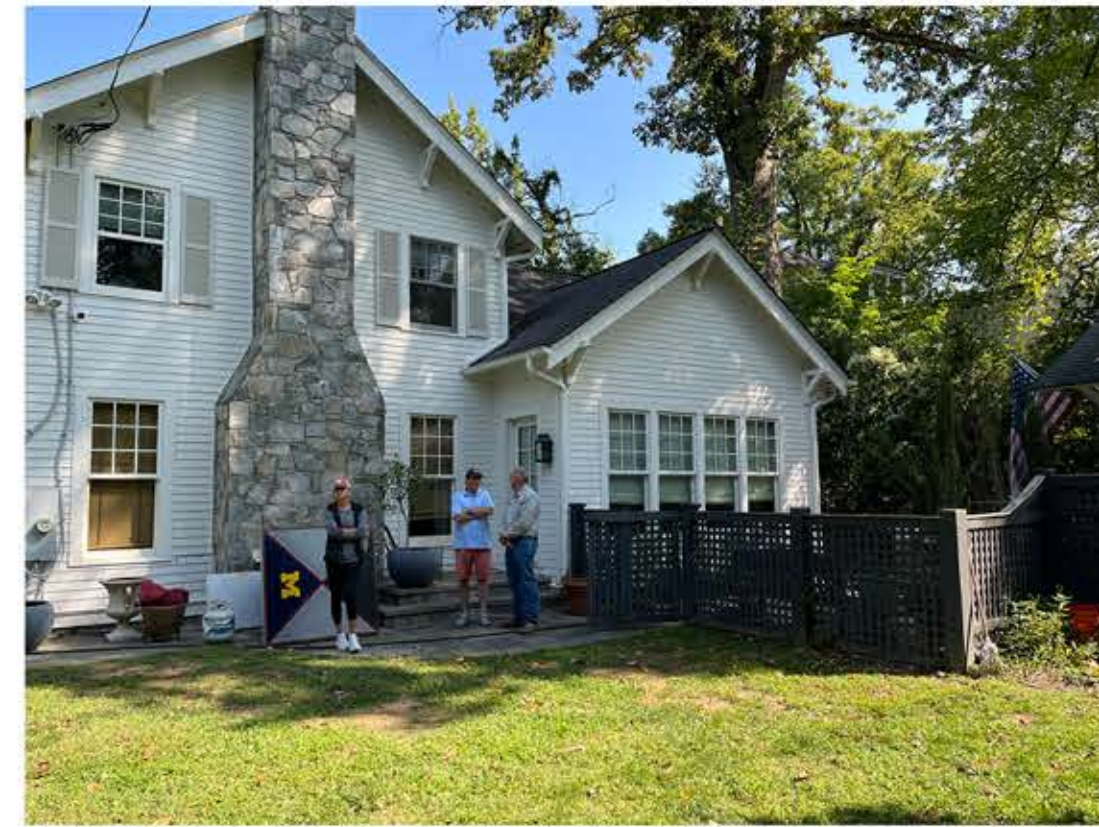
View of the Rear of House. Proposed stone facade will match the chimney
