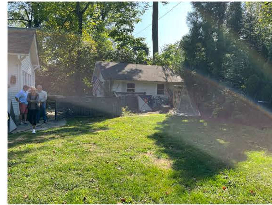
View of the Detached Garage and Rear Screen Plantings
