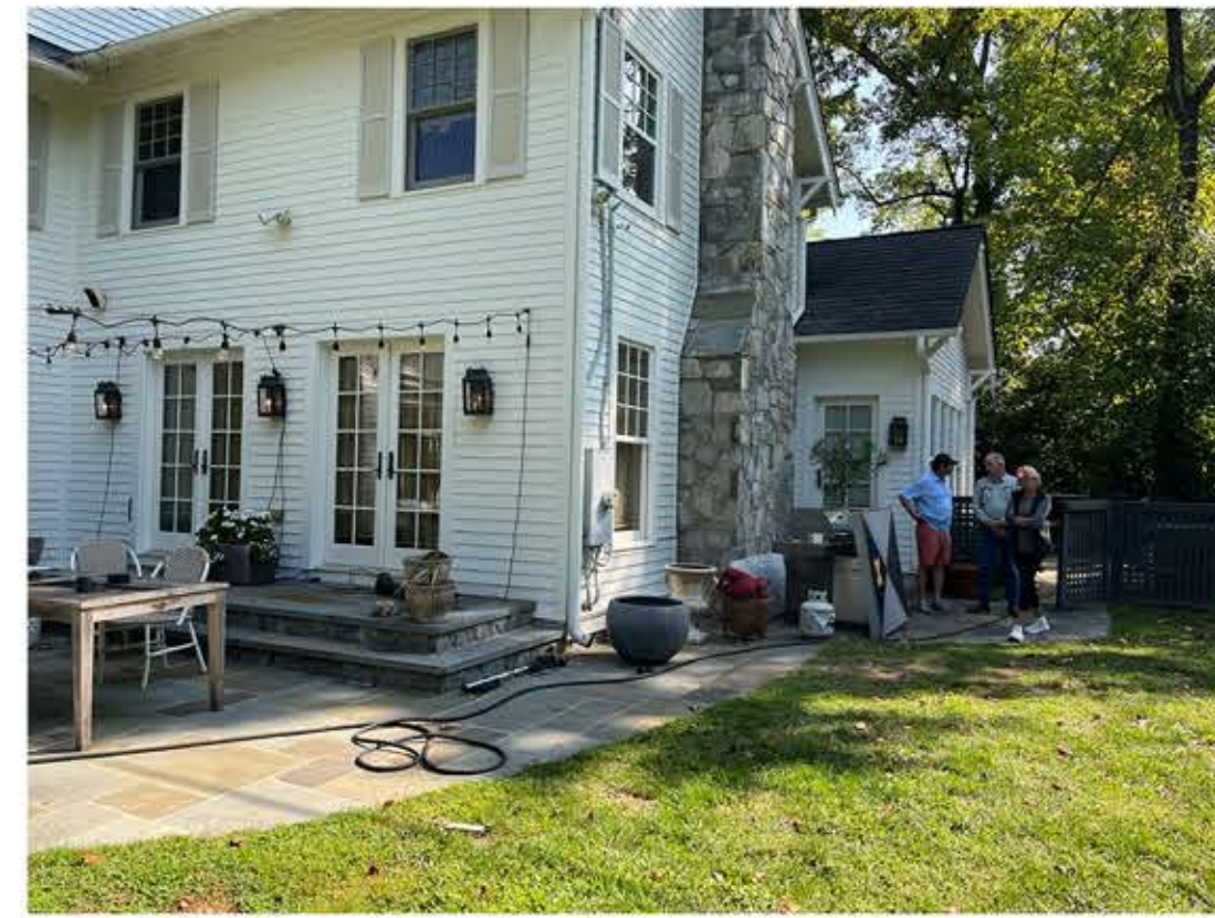
View of the existing Patio/ Walkway and Rear of House
