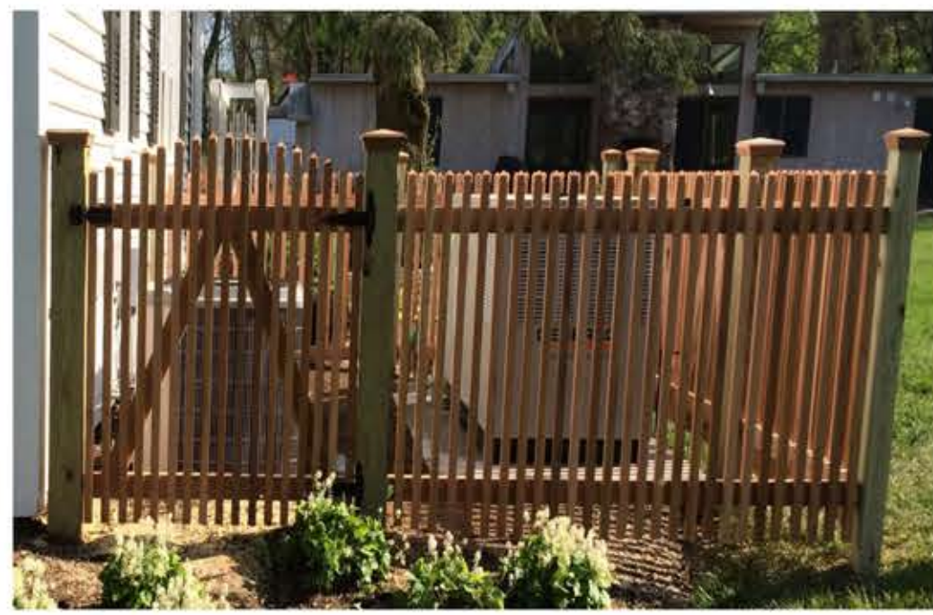
5' height Cedar Picket Fence w/ Cedar Posts and Caps (Pressure Treated Posts to be wrapped in Cedar). No staining or painting proposed. Gate pickets to be level to match fence pickets.
