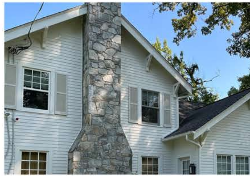
Dove Grey Natural Stone, as found on existing Chimney
