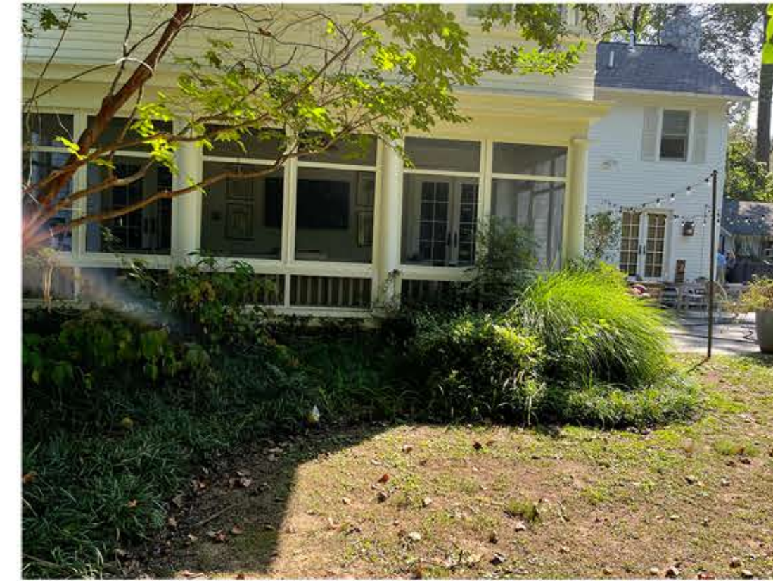
View of the side of the Screened Porch
