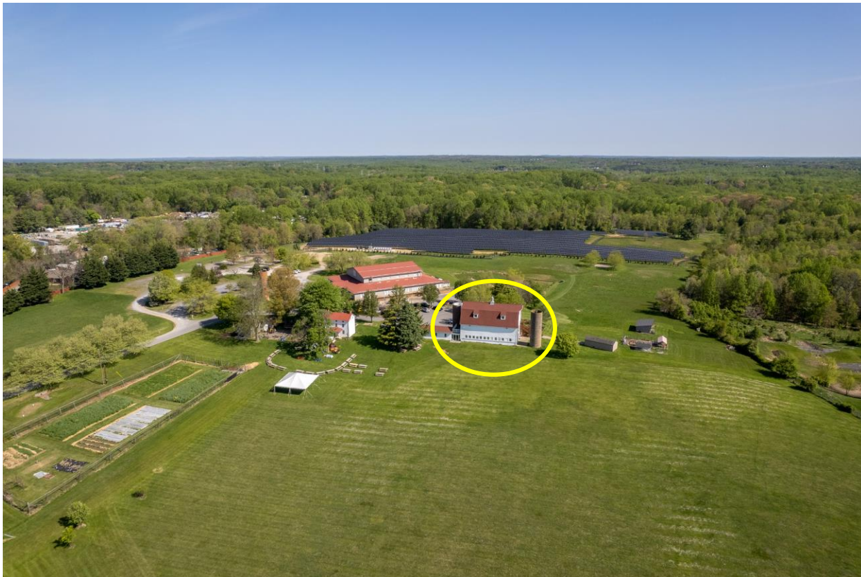
Figure 5: Aerial photograph of the Spencer-Carr Master Plan site with the rehabilitated dairy barn and its silos circled in yellow.
