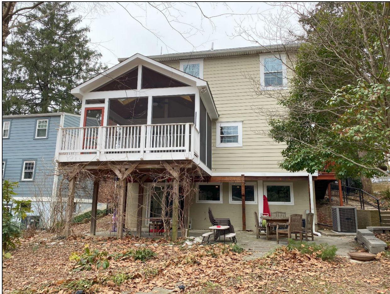
Figure 3: Rear view of subject property (Montgomery County Planning Staff, 2025).
