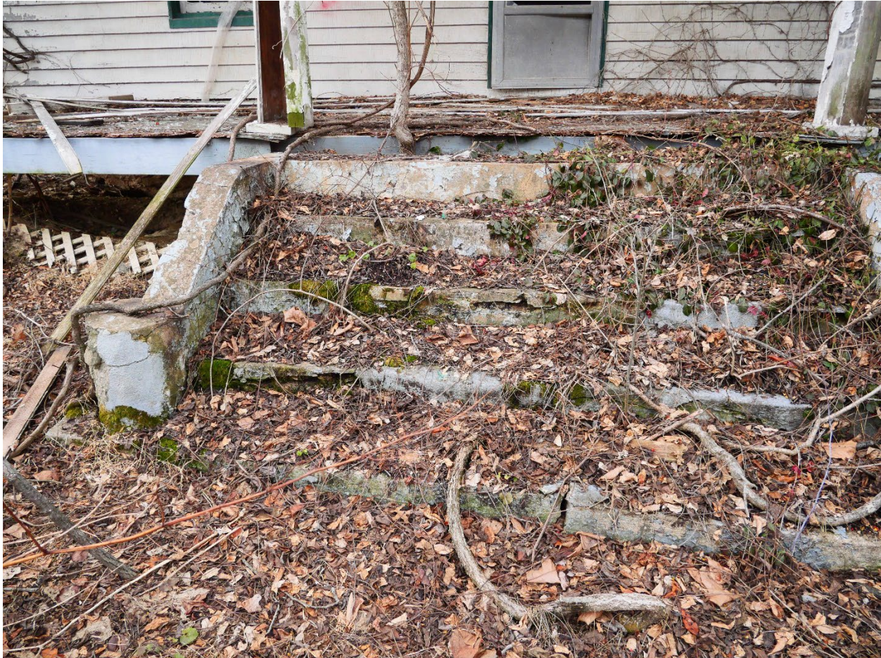
Figure 26: Close up of conditions of porch, Montgomery Planning, 2025.
