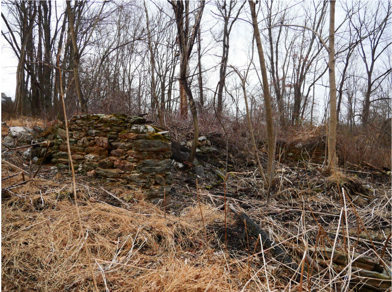
Figure 45: Extant corner of demolished bank barn, Montgomery Planning, 2025.
