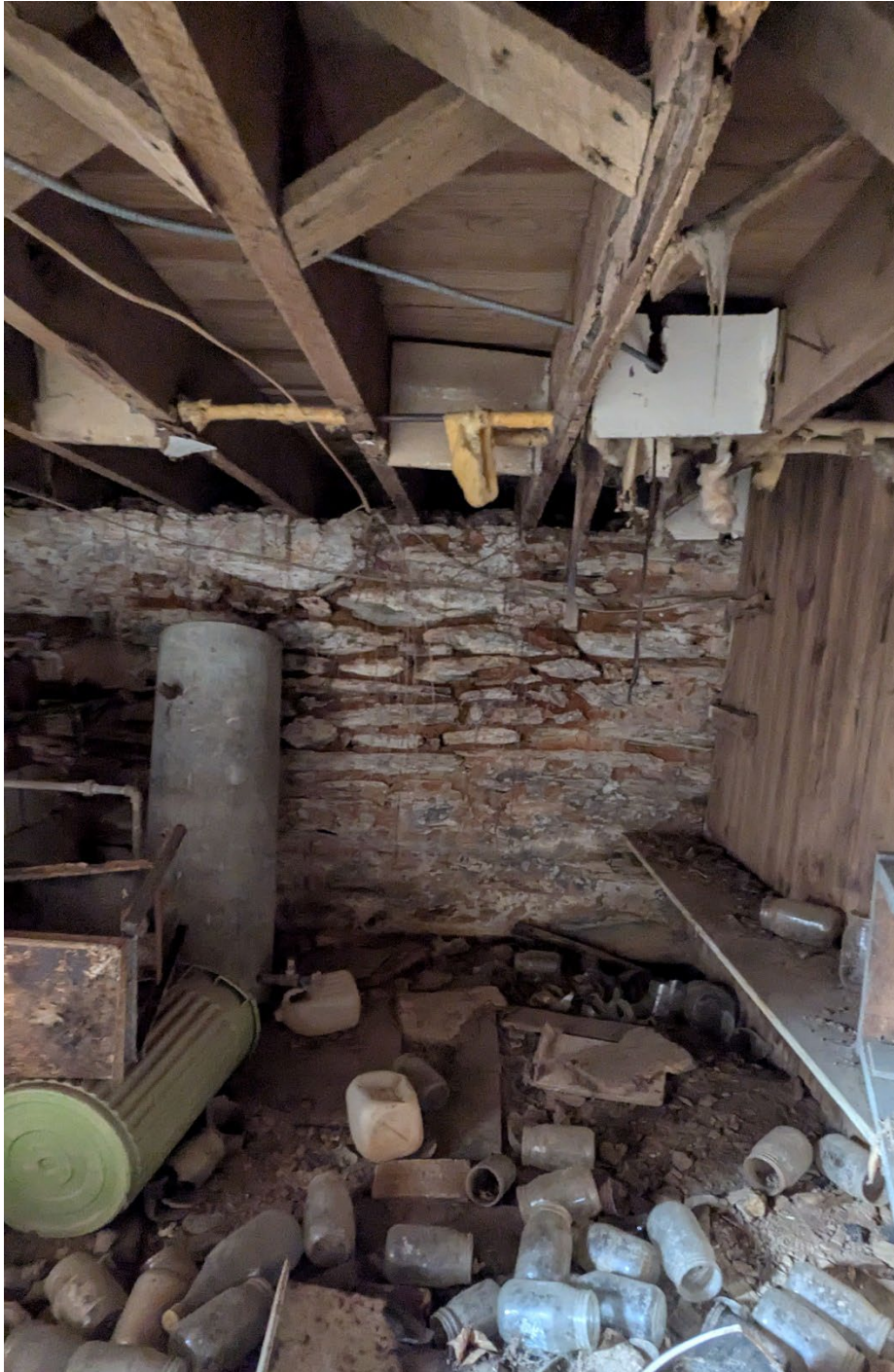
Figure 23: Interior of cellar, Montgomery Planning, 2025.
