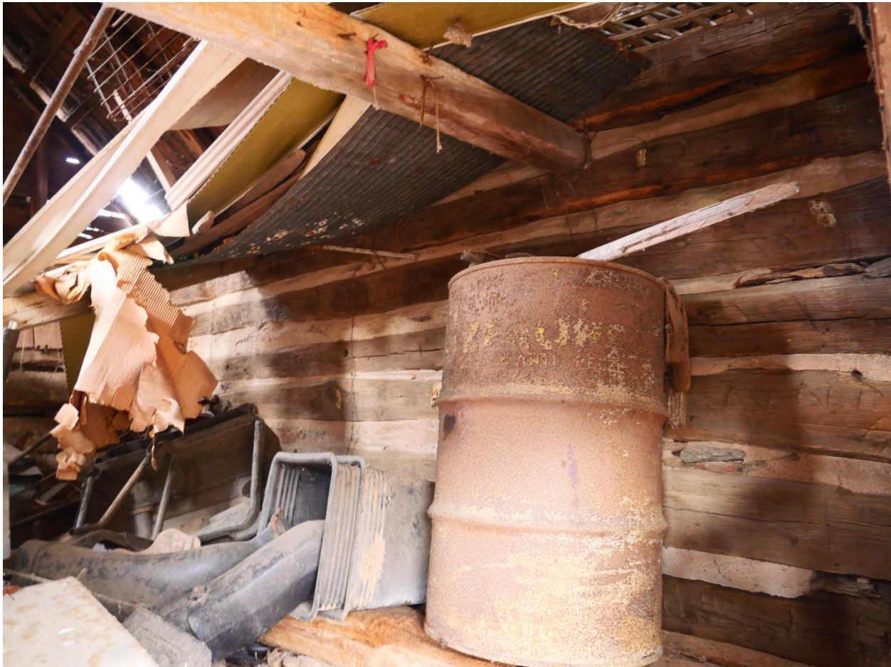
Figure 40: Interior of log shed, Montgomery Planning, 2025.
