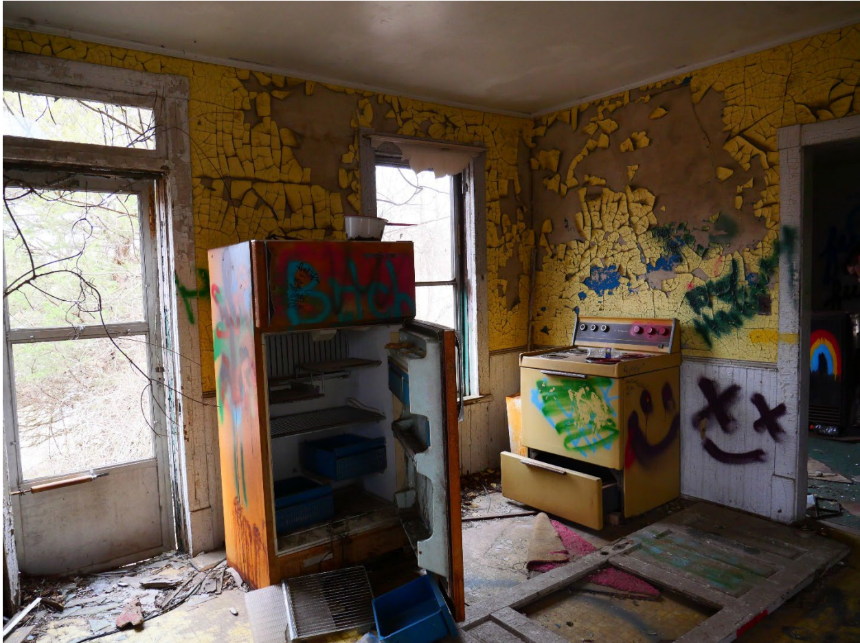
Figure 32: Conditions of kitchen wing, Montgomery Planning, 2025.
