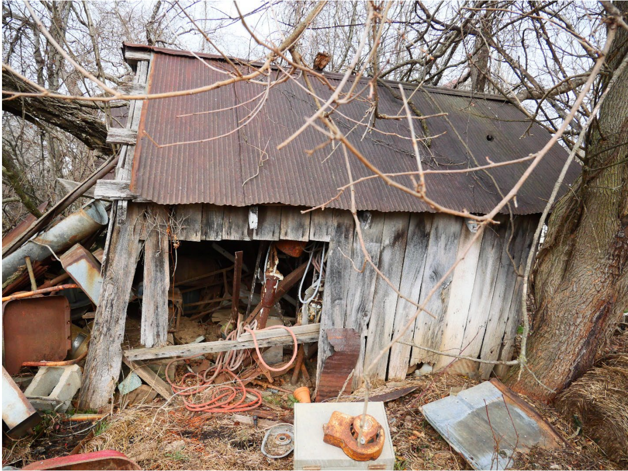
Figure 44: View of rear elevation of frame shed, looking east, Montgomery Planning, 2025.
