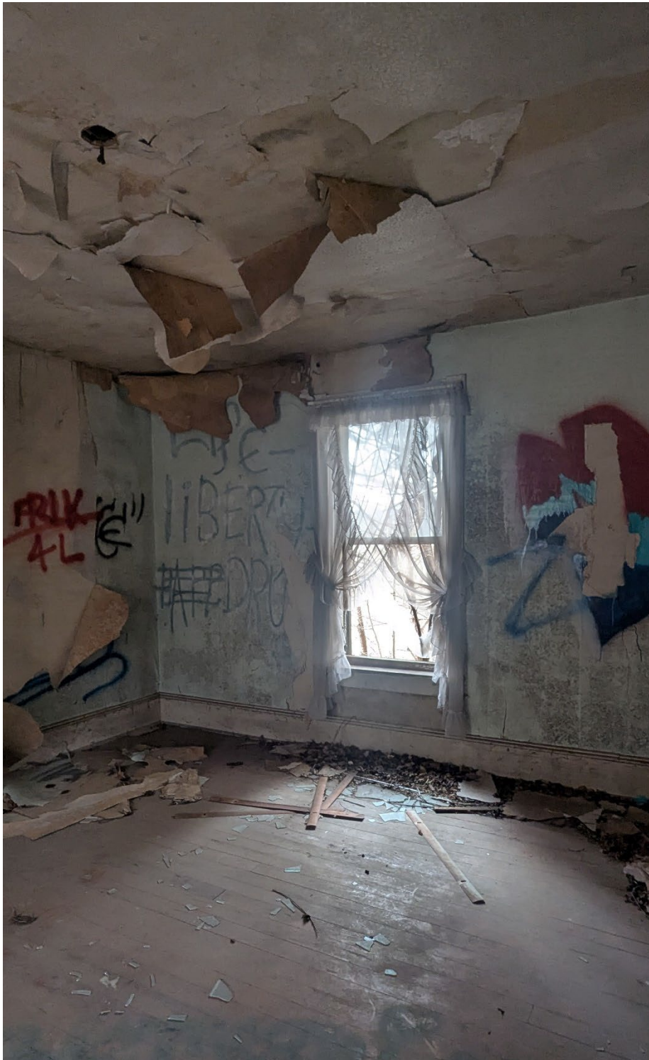
Figure 34: Conditions of living room, Montgomery Planning, 2025.
