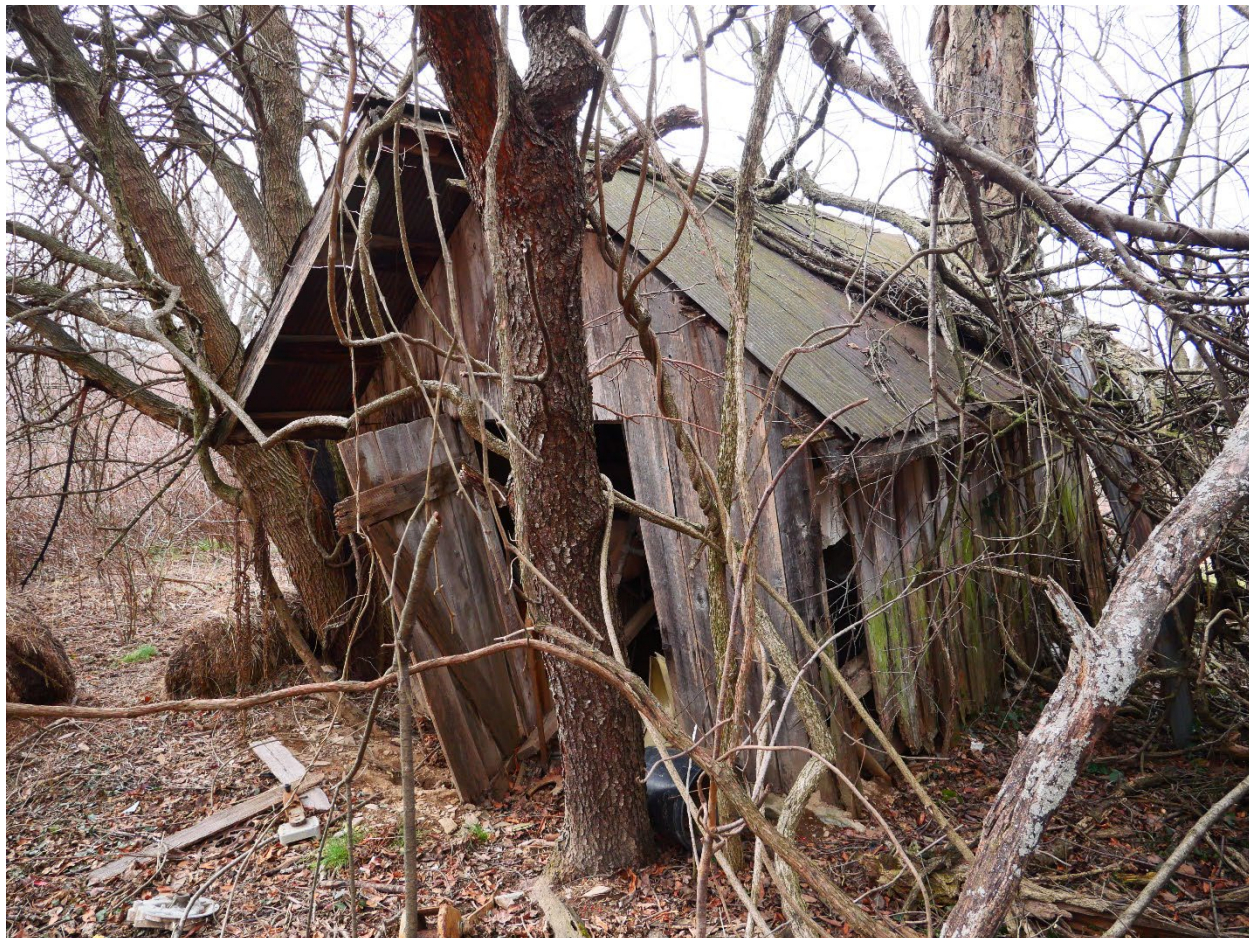
Figure 43: View of frame shed, looking southwest, Montgomery Planning, 2025.
