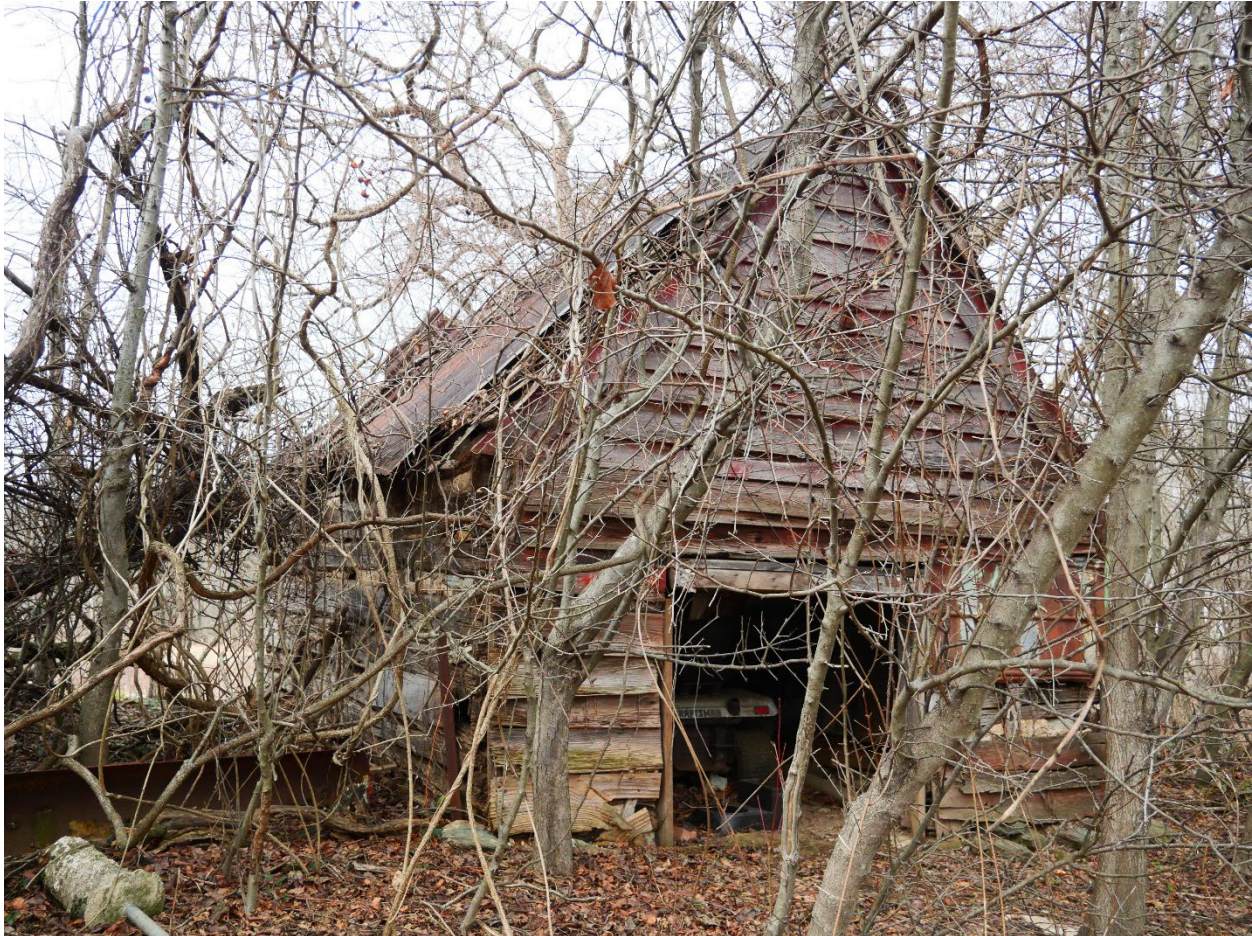
Figure 38: View of log shed, looking northwest, Montgomery Planning, 2025.
