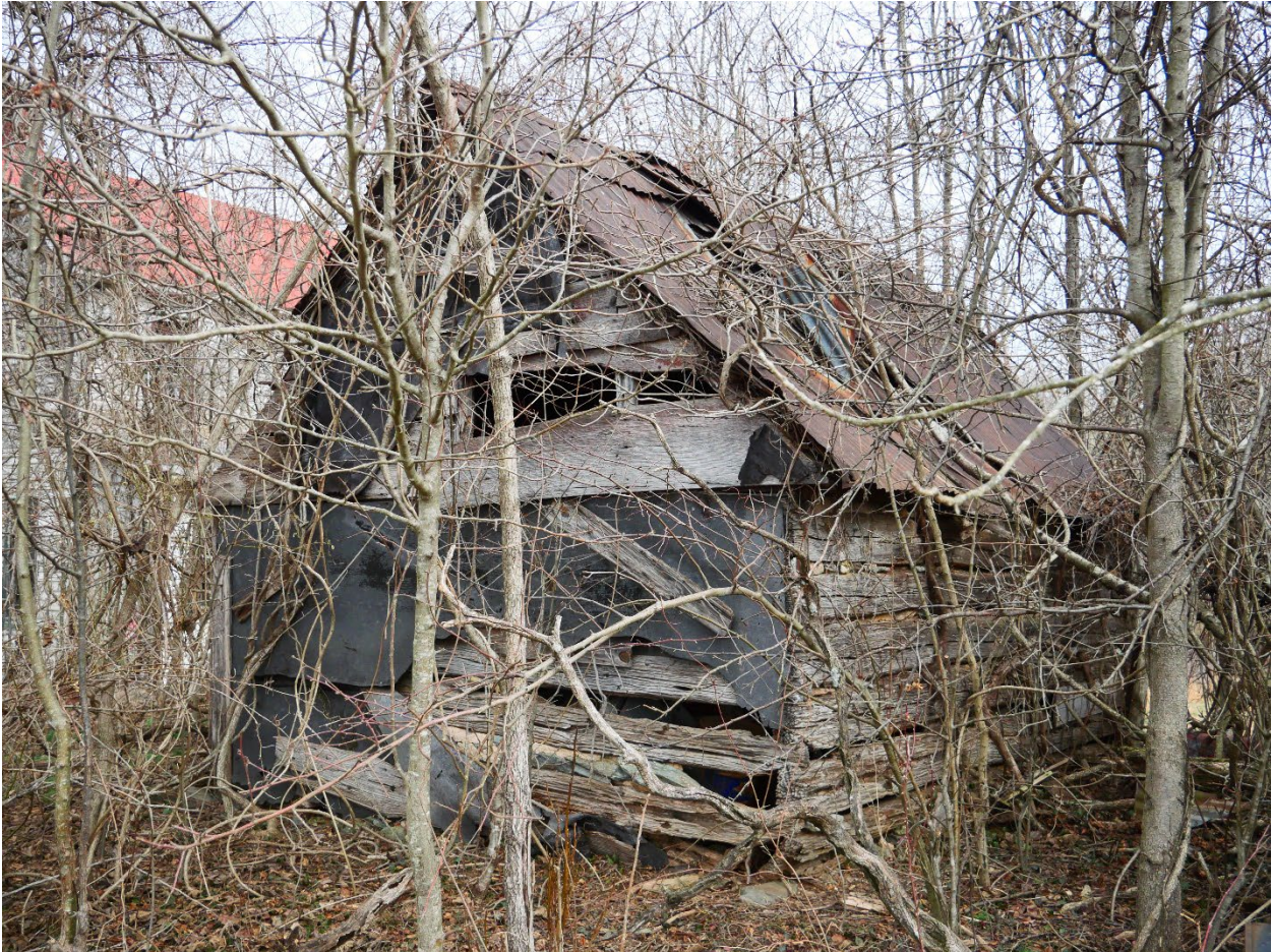
Figure 39: Rear of log shed, Montgomery Planning, 2025.
