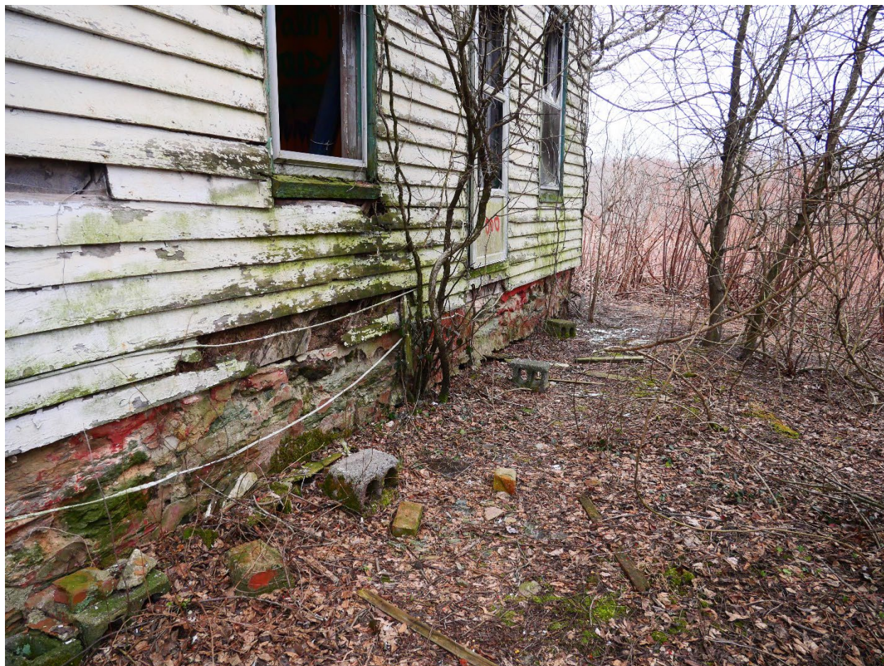
Figure 27: Close up of conditions of north side, Montgomery Planning, 2025.
