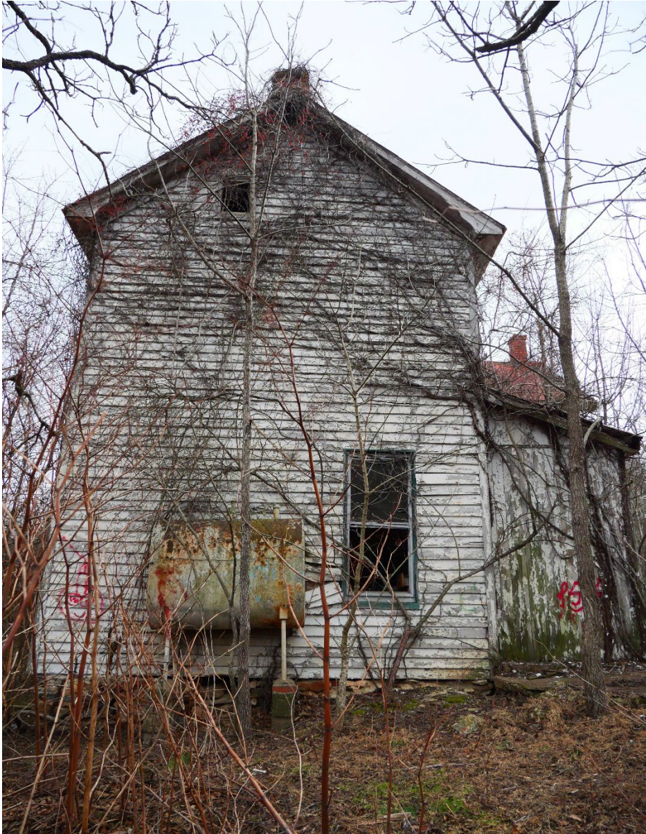
Figure 20: View of west elevation of the Charles M. King farmhouse, Montgomery Planning, 2025.
