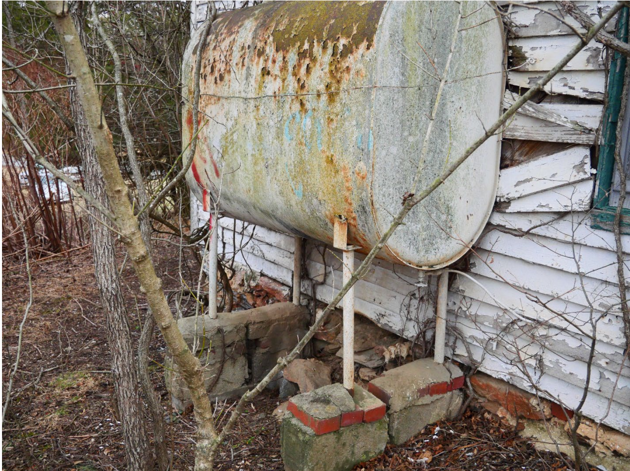
Figure 28: Close up of conditions of west side of farmhouse, Montgomery Planning, 2025.
