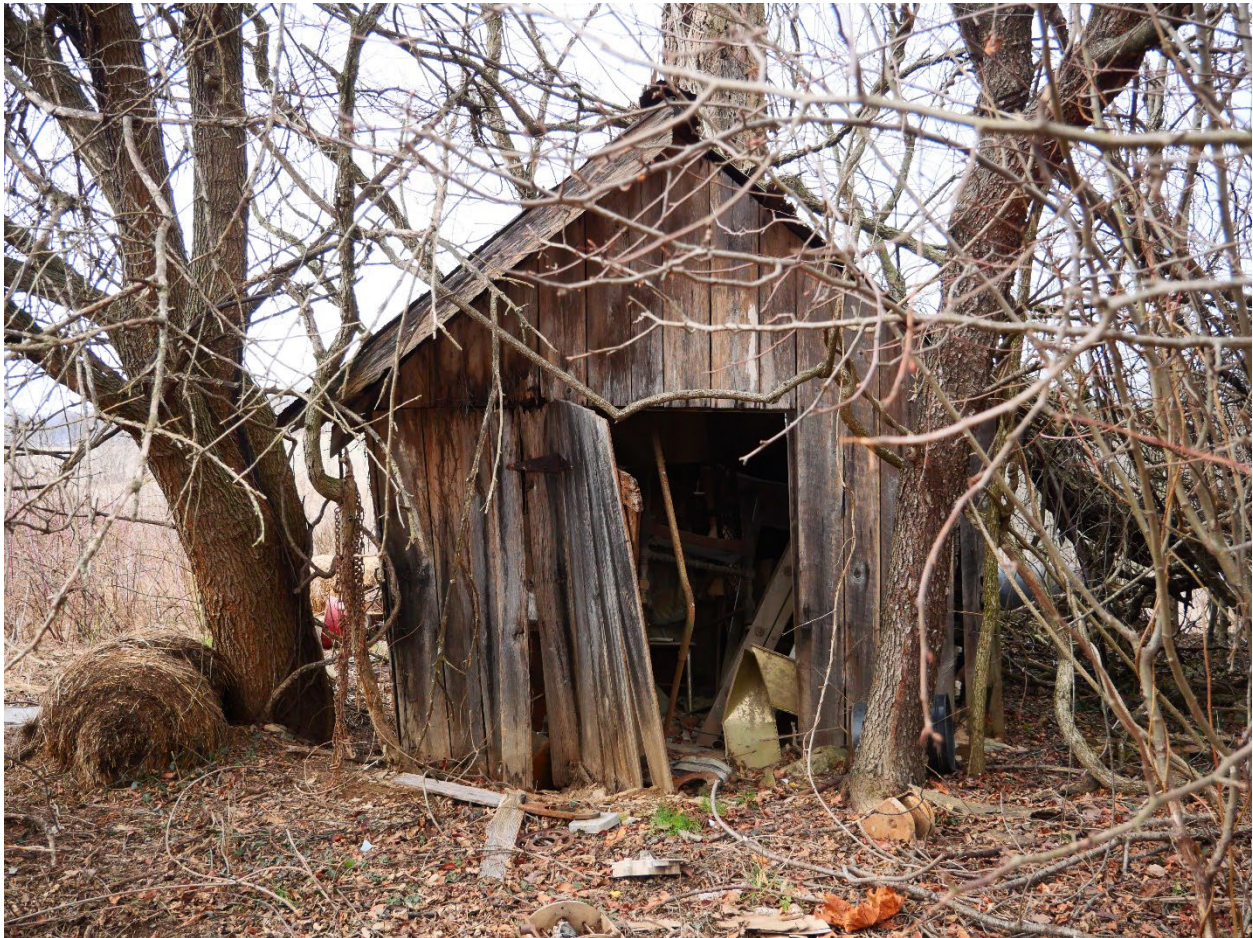
Figure 41: View of east elevation of frame shed, Montgomery Planning, 2025.
