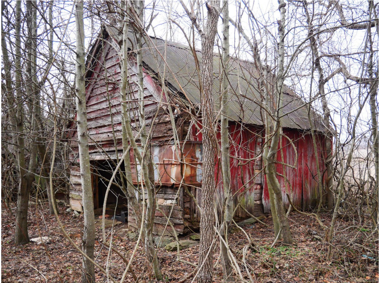
Figure 37: View of log shed, looking southwest, Montgomery Planning, 2025.
