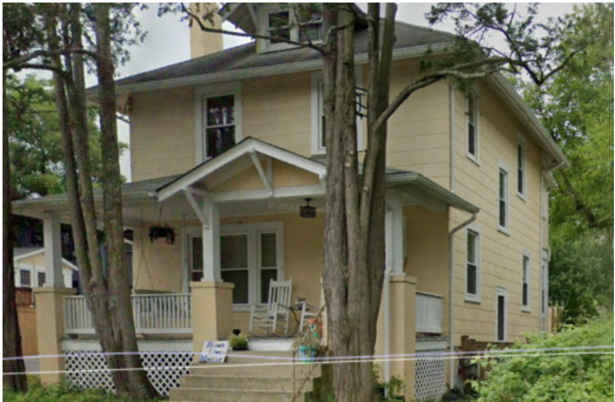
AFTER --- CURRENT VINYL WINDOWS - INSTALLED IN 2014
