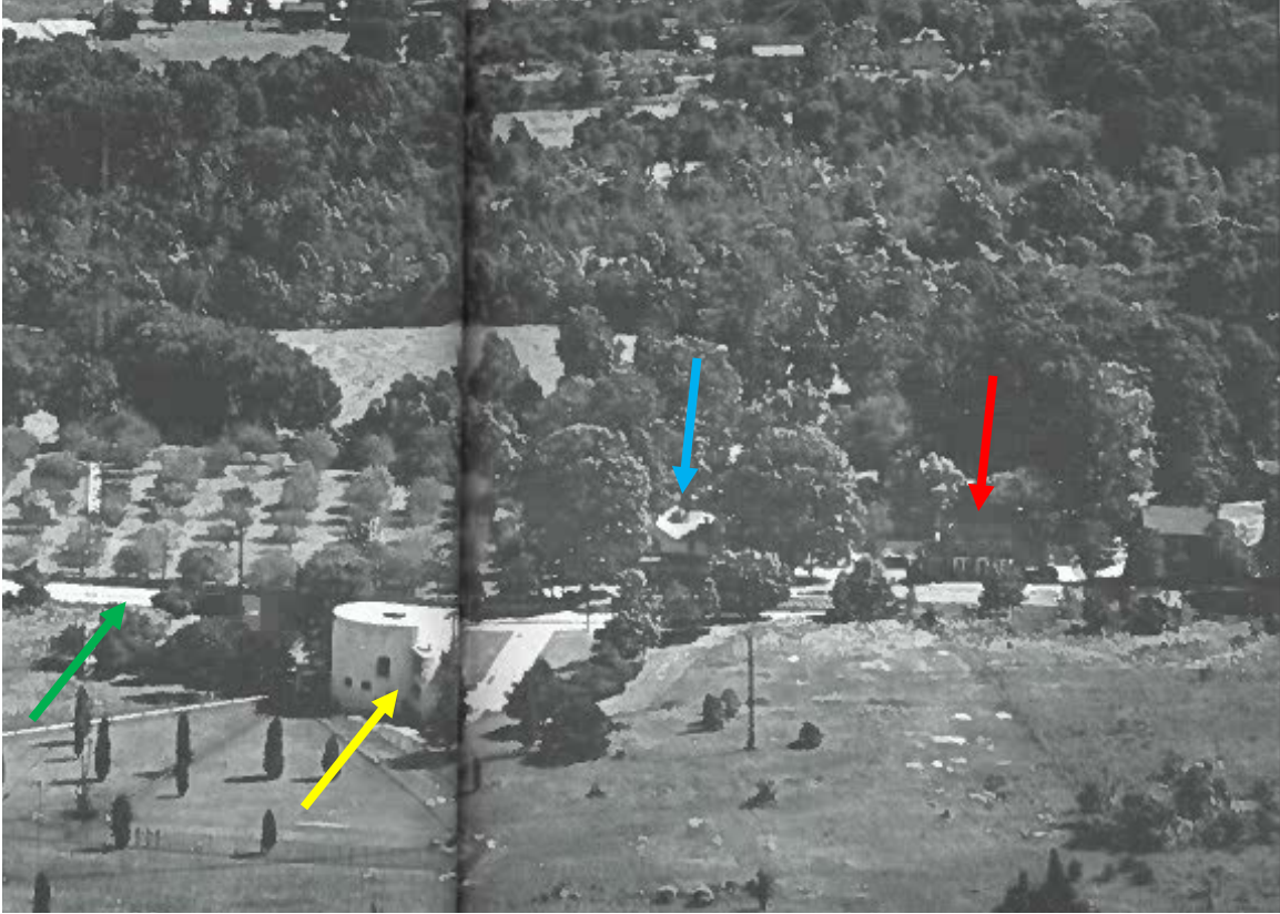
Figure 1: Aerial photograph, 1948. The yellow and green arrows point to the WTOP Radio Station and Old Bladensburg Road—present day University Boulevard West—in the foreground, respectively. The red and blue arrows point to the Romeo and Elsie Horad House and the demolished Charles and Jane Webster House in the background, respectively. The family fruit orchard is visible in the midground on the left.
