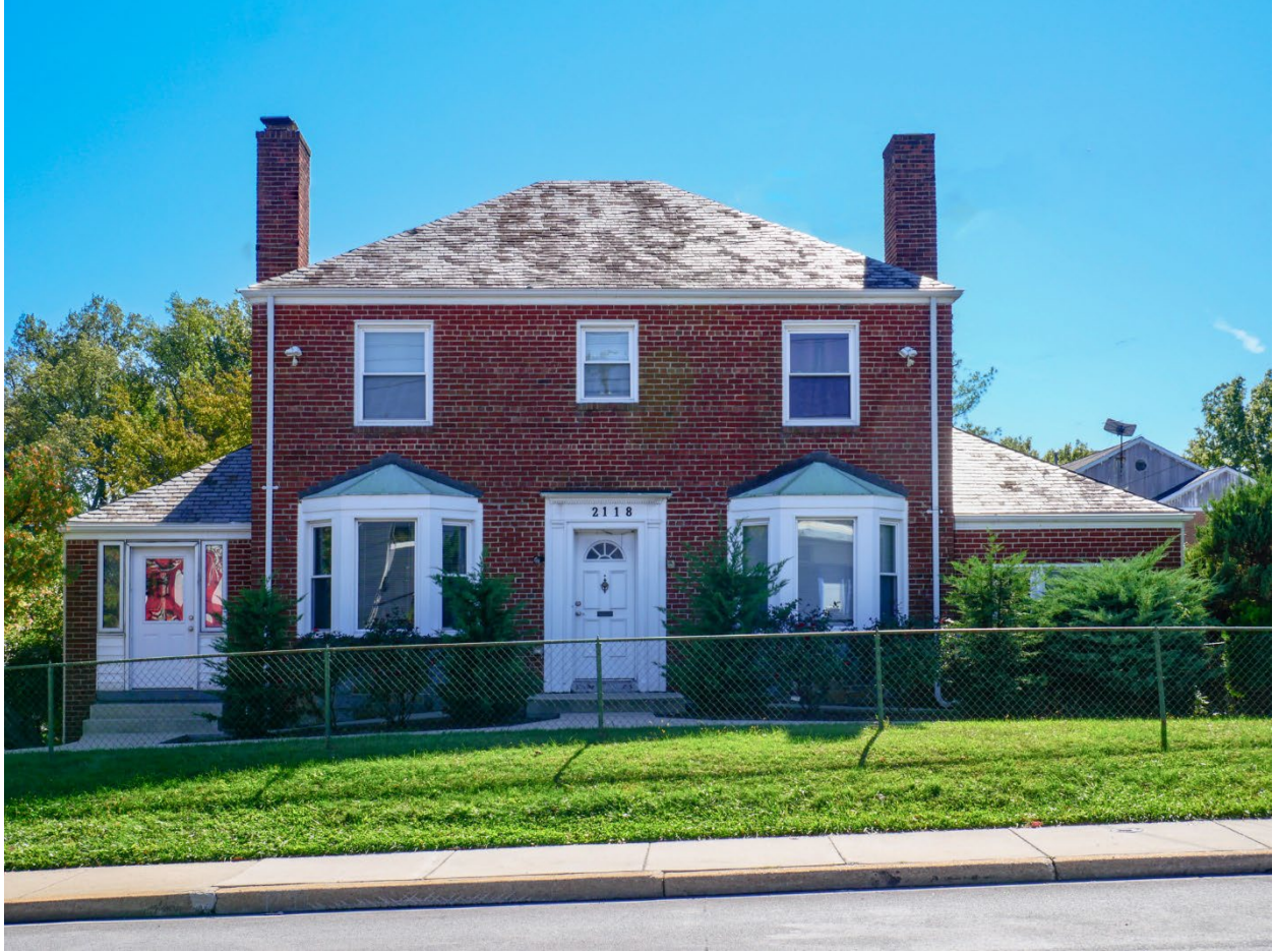
Figure 1: View of the façade of the Romeo and Elsie Horad House looking south from University Boulevard West, 2022.
