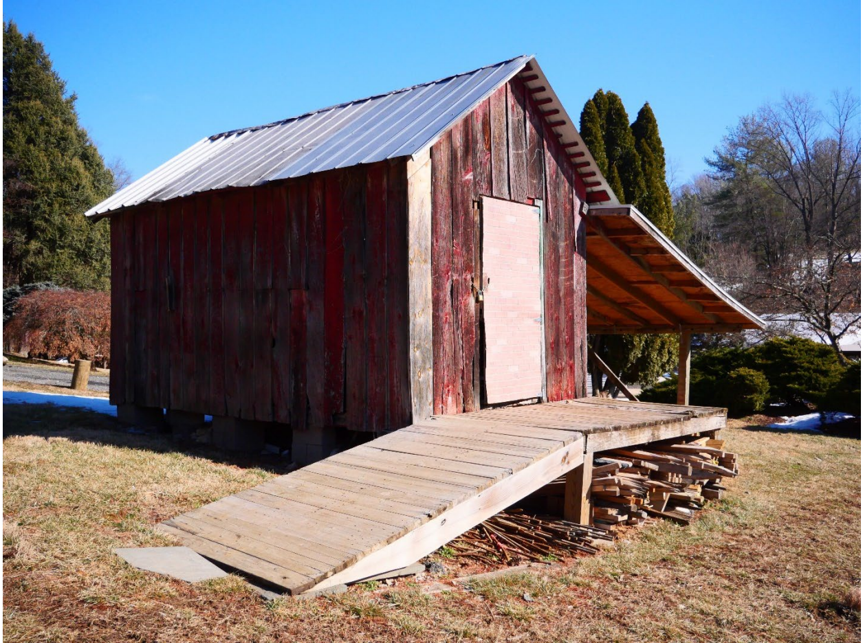
Figure 17: View of the early twentieth century outbuilding, 2025. Source: Montgomery Planning.
