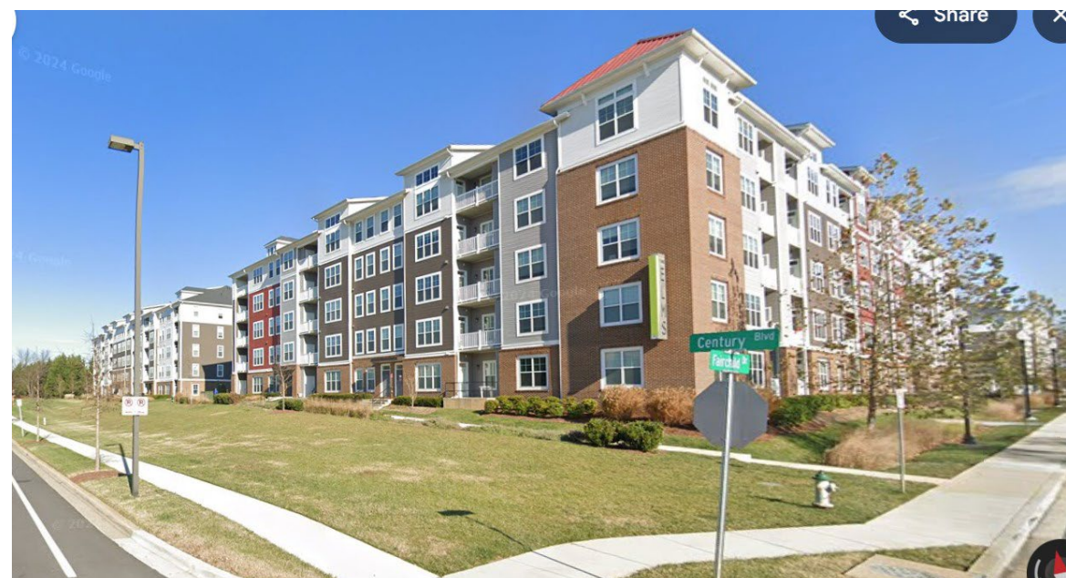
Apartments - Cloverleaf Development
