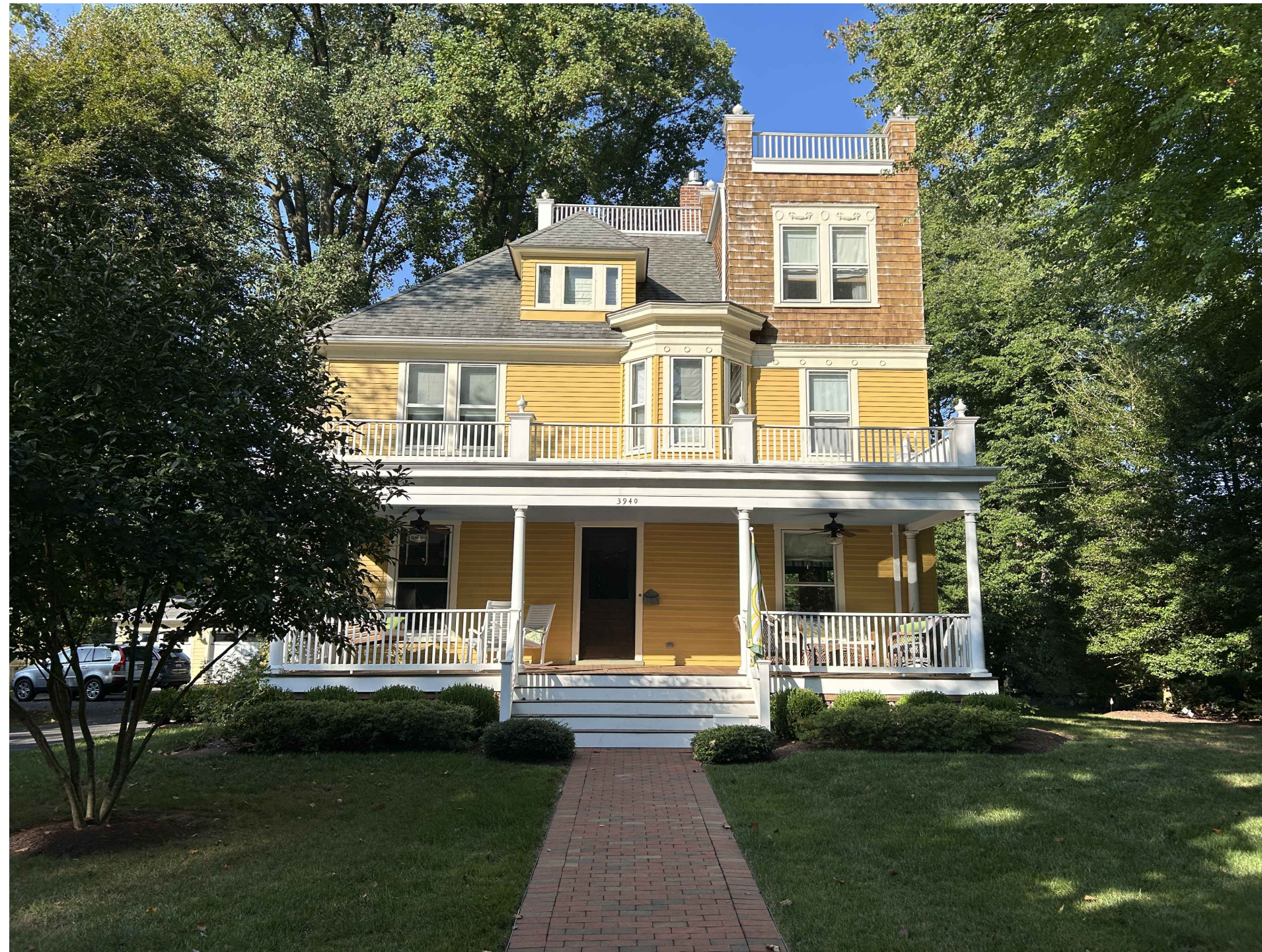
EXISTING 3 STORY FRAME HOUSE (FRONT VIEW)
