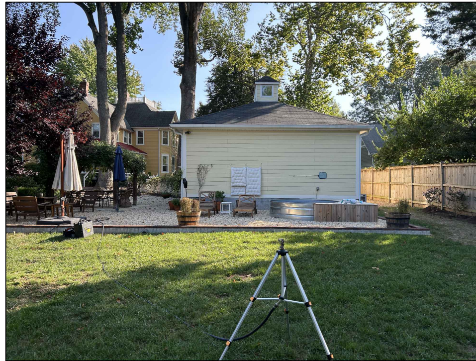
EXISTING 1 STORY GARAGE (FRONT VIEW)
