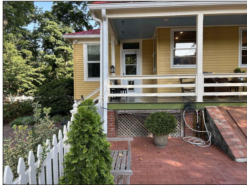
EXISTING 3 STORY FRAME HOUSE (LEFT SIDE)
