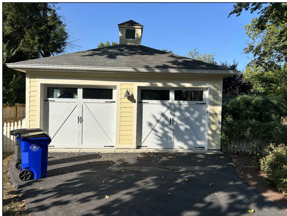
EXISTING 1 STORY GARAGE (FRONT VIEW)
