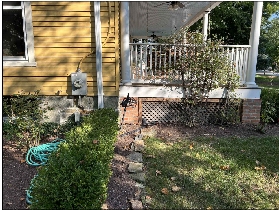
EXISTING 3 STORY FRAME HOUSE (LEFT SIDE)
