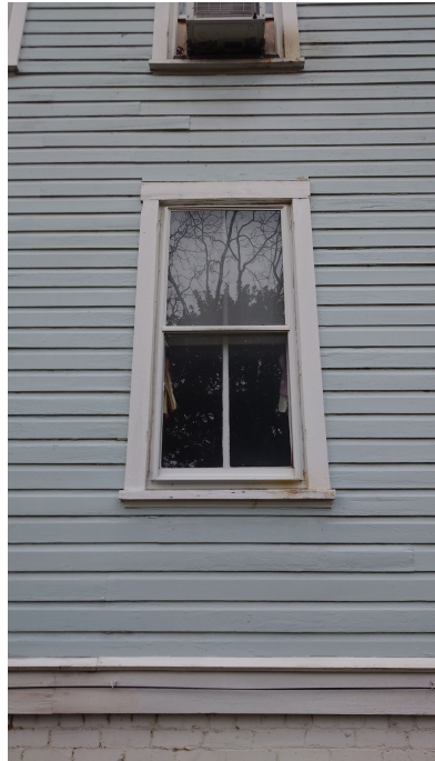
Window Detail Photo Painted wood double hung with aluminum storm windows
