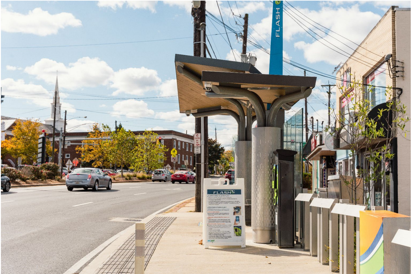
Flash BRT Station
