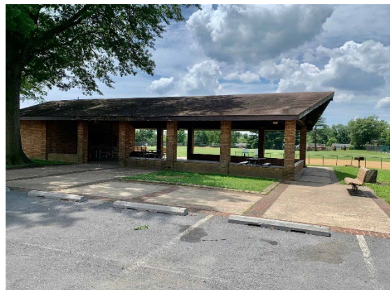
Wheaton Forest Local Park Picnic Shelter
