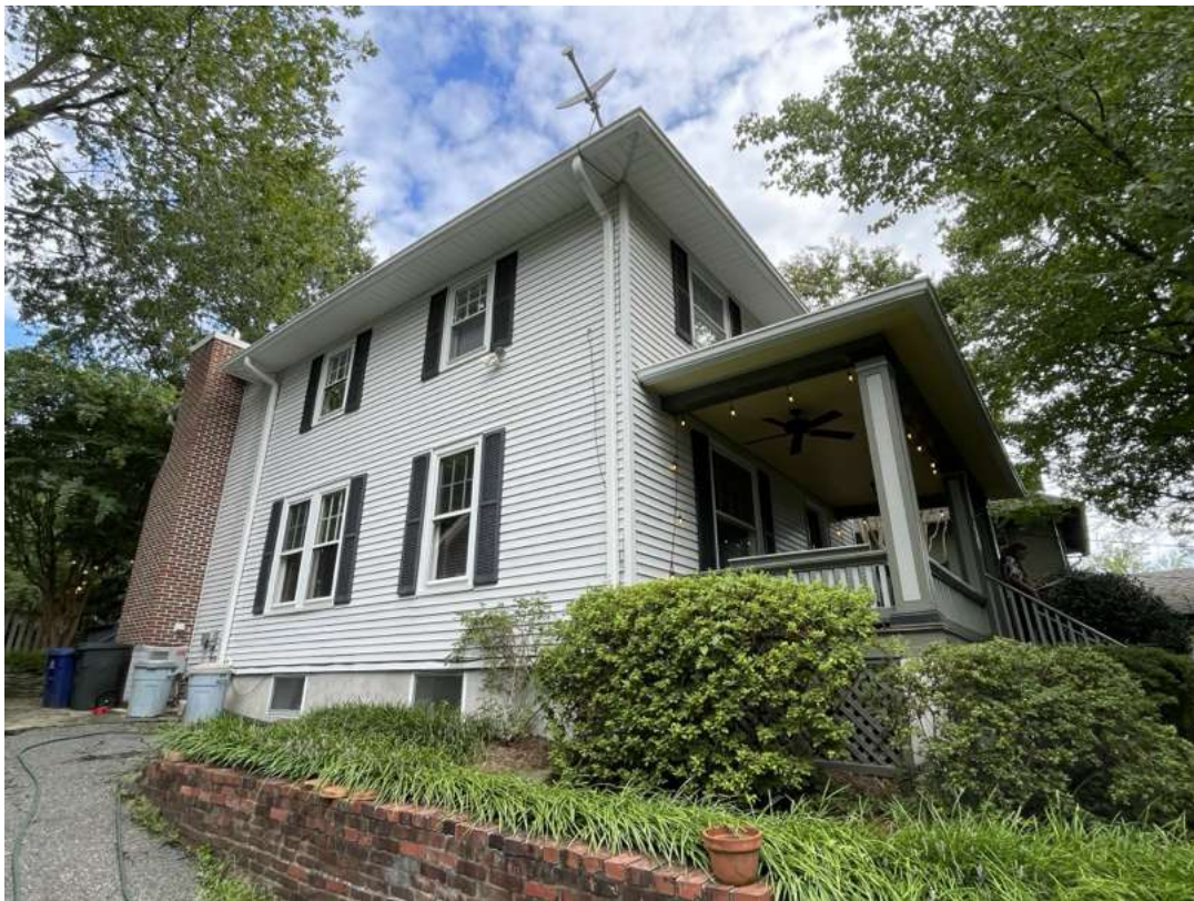
Detail: 30 COLUMBIA AVE. WEST CORNER
