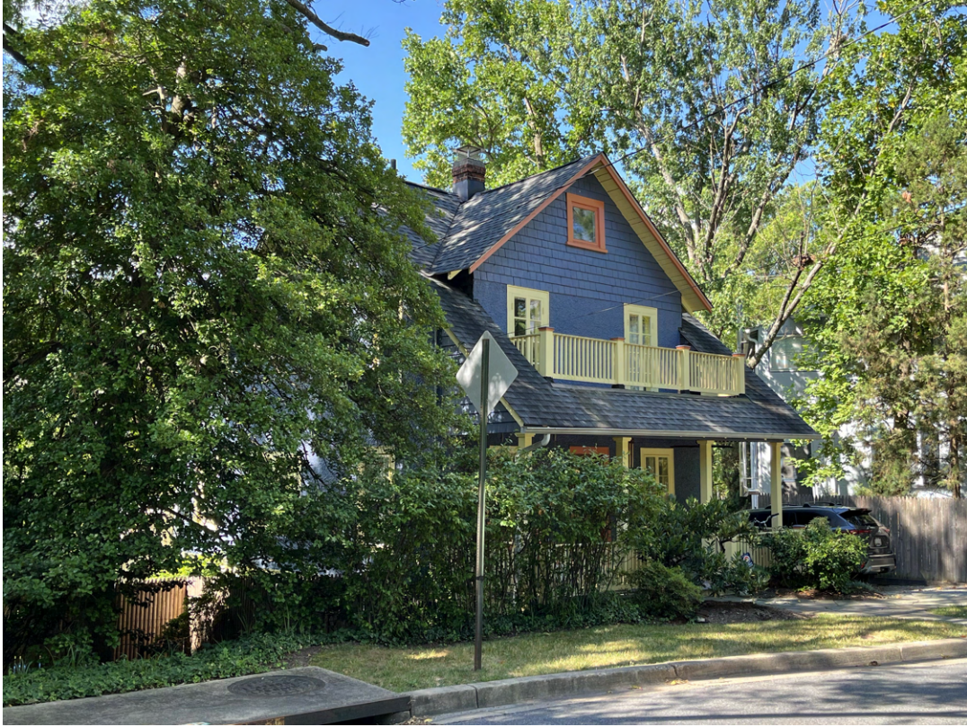
Detail: 51 ELM AVE. APPROACH FROM EAST
