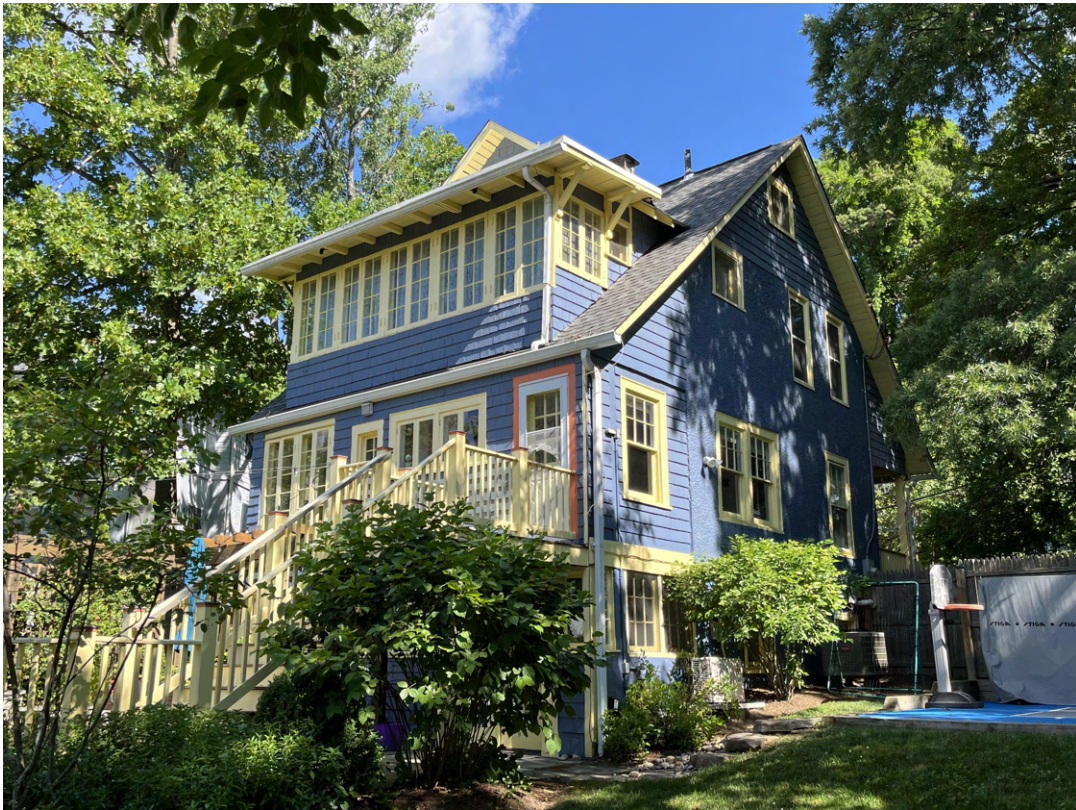
Detail: 51 ELM AVE. SOUTH-EAST CORNER
