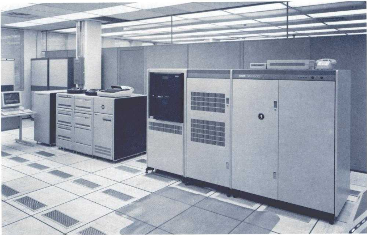
Figure 3. The master control station is the focal point for mission and experiment operations
