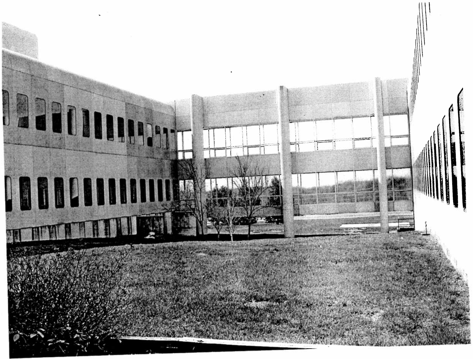
fig. 15. Photograph from the central spine through the landscape to the catwalk, COMSAT Laboratories (Cesar Pelli for DMJM architect), Clarksburg, MD, taken 2002. Source: Mary Corbin Sies
