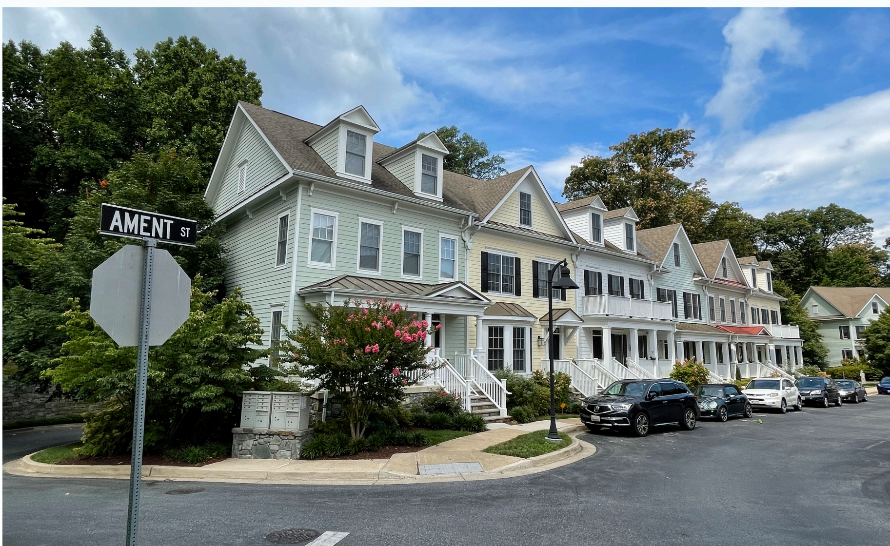
Porches and stoops add architectural detail to the fronts of townhomes
