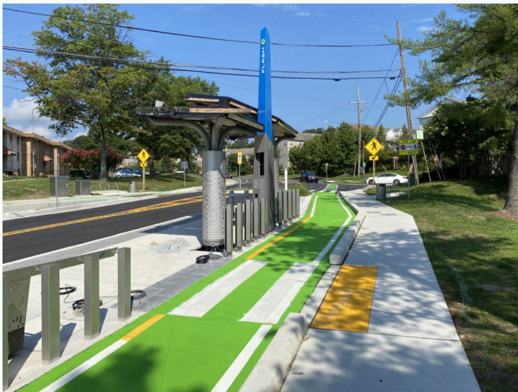
A BRT station on the US 29 BRT Flash route
