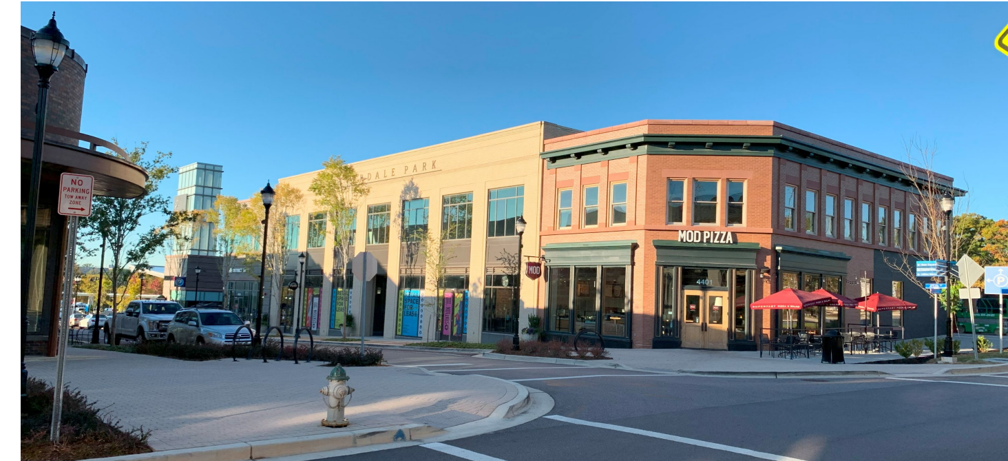
Retail fronting streets with parking behind at the Riverdale Park Town Center
