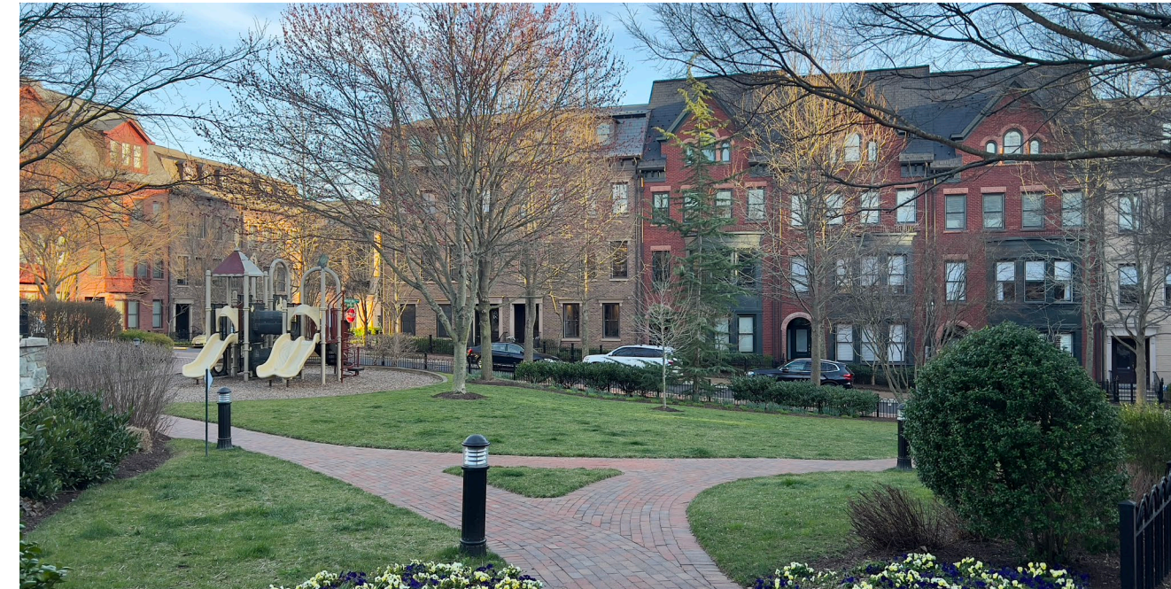
Small residential green with homes facing the green at Park Potomac
