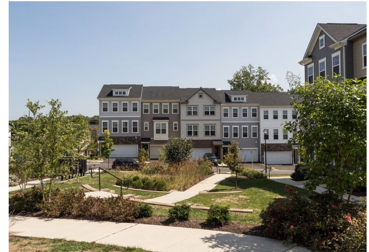
Stormwater management facilities in a common space at Dowden's Station neighborhood
