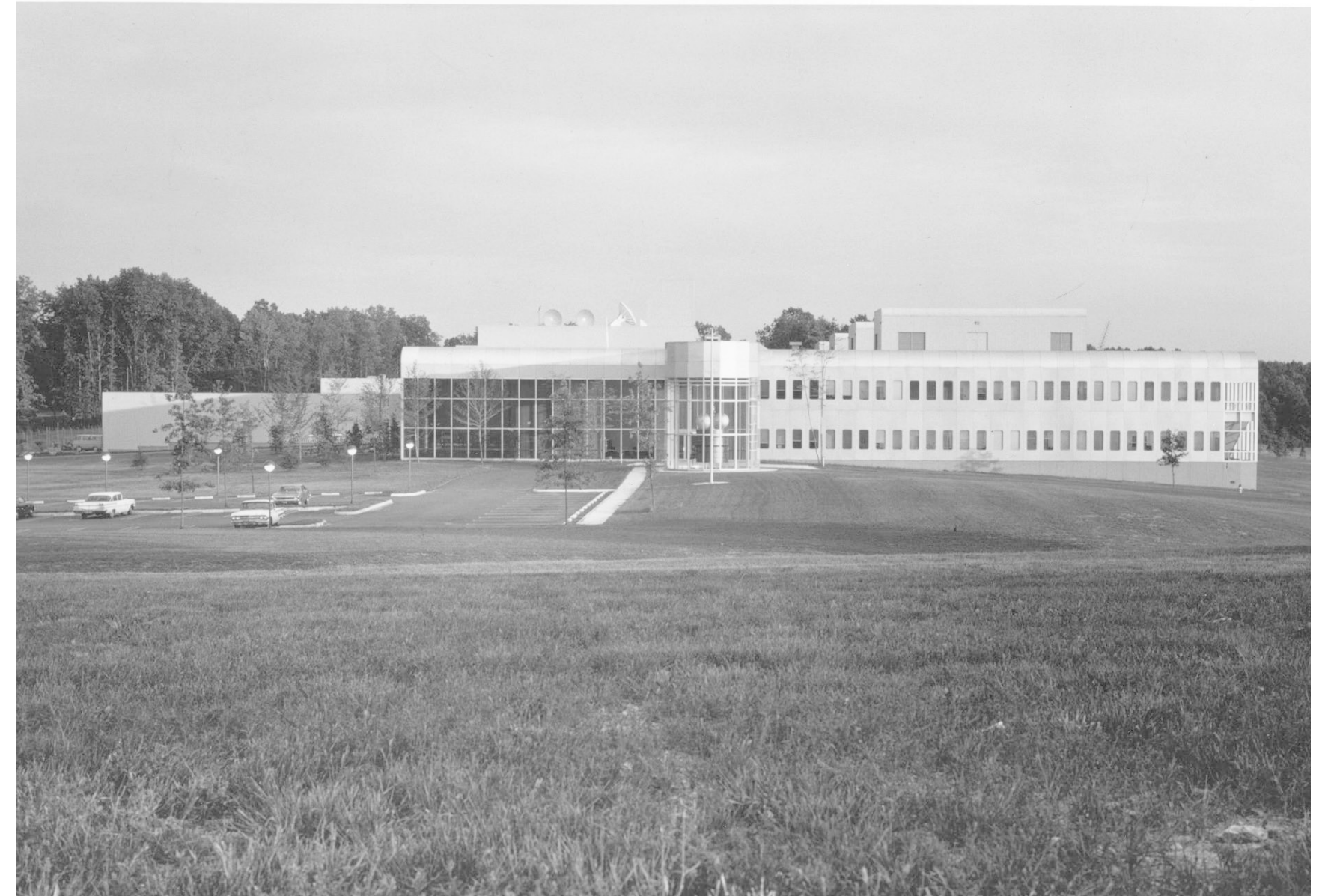
View of the north elevation of COMSAT Laboratories, ca. 1969. Source: Montgomery Planning Archives.
