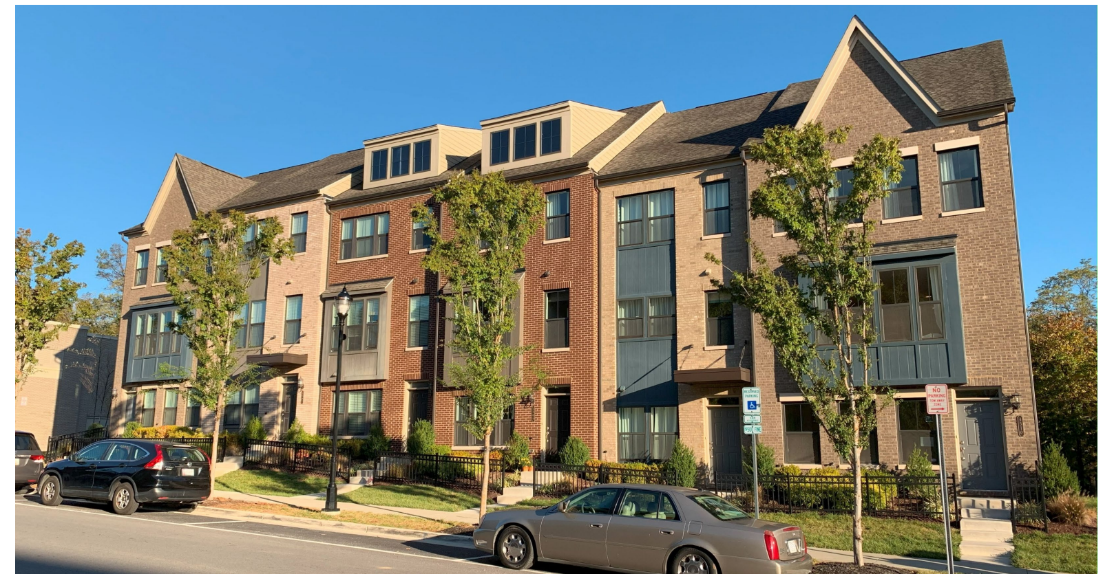
Composition of a townhouse string at the Riverdale Park Town Center
