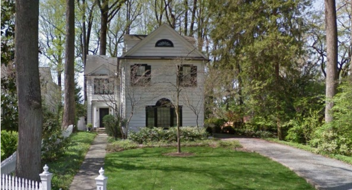
Figure 4: 5914 Cedar Parkway was constructed in 1923.
