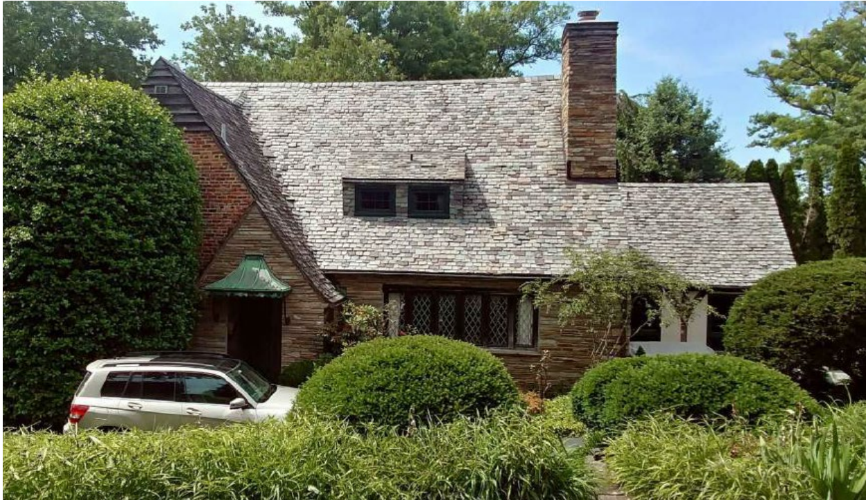
Figure 8: Existing front elevation of the subject property.
