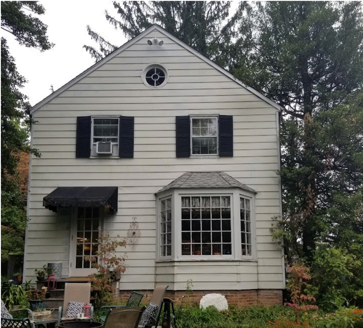
South side of the house
