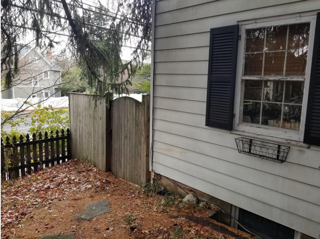
Existing solid wood fence gate from the north
