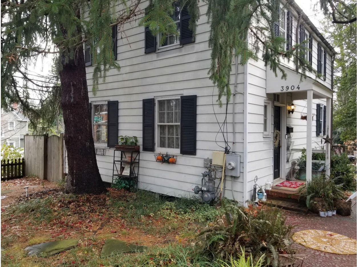
North side of the house, including Pepco electric meter and Verizon ONT
