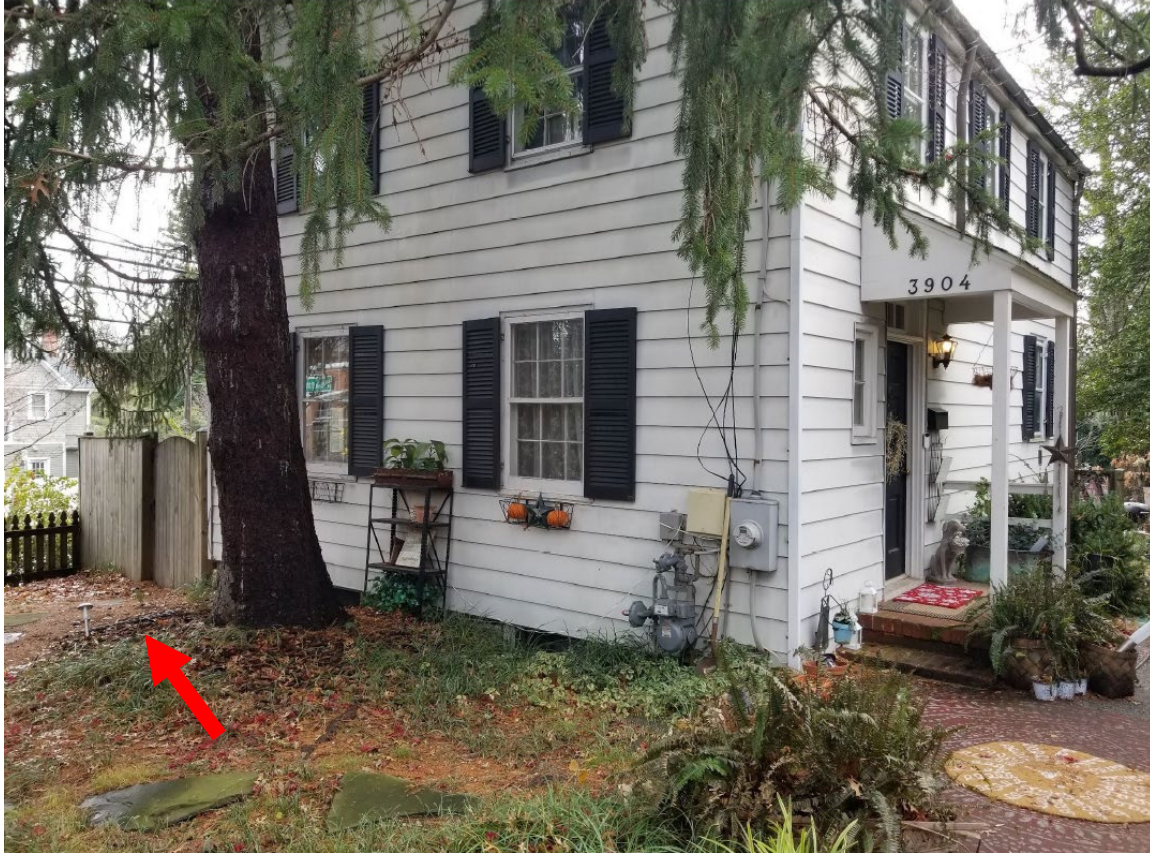
Figure 5: View of the Washington Street elevation of the subject property. A red arrow points to the location of work.
