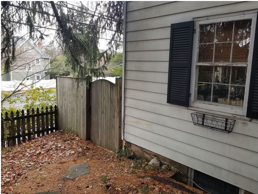
Figure 4: Closer view of the area of work. The proposed fence extension will match the existing privacy fencing in materials and appearance.
