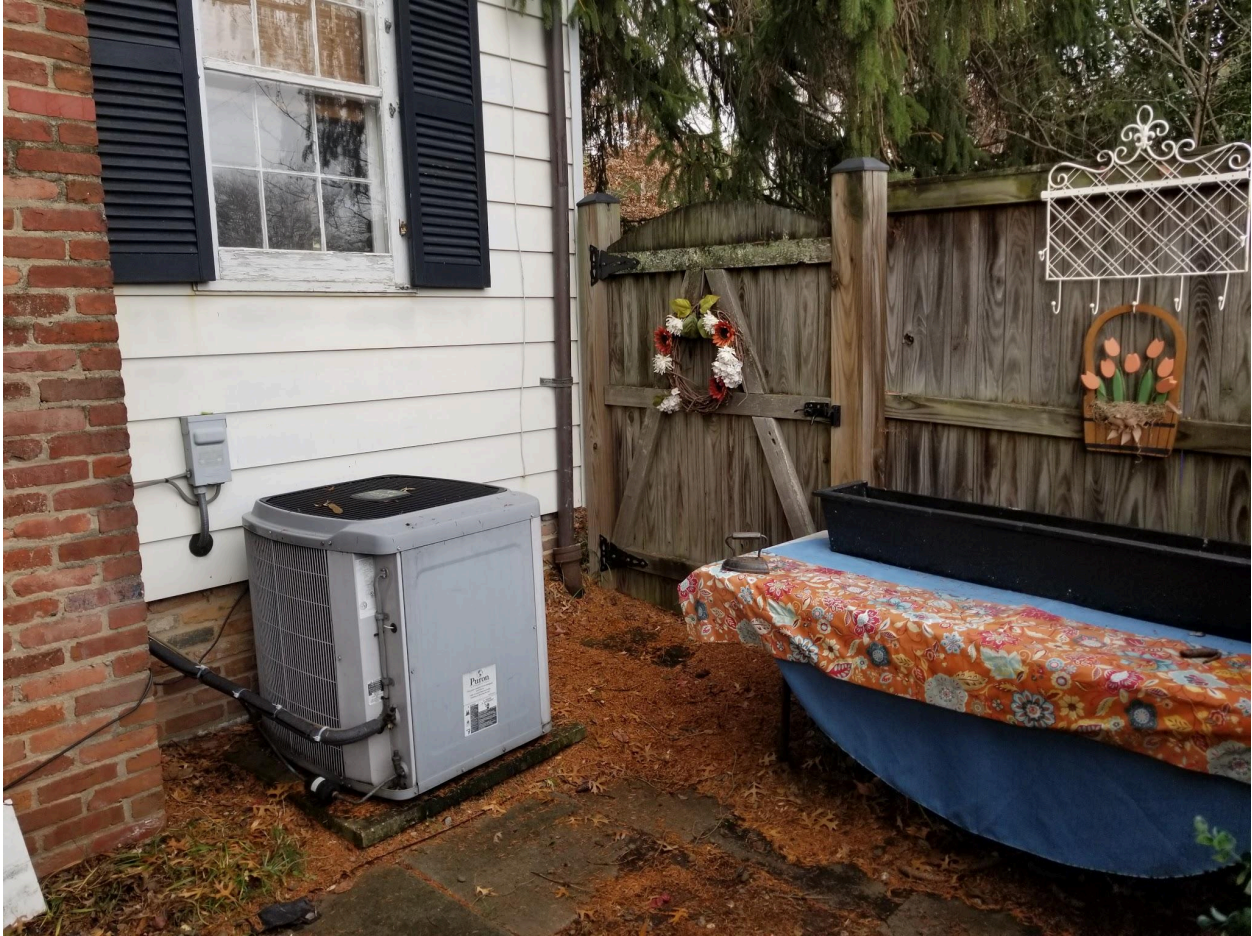
Existing fence gate and air conditioning compressor from the south
