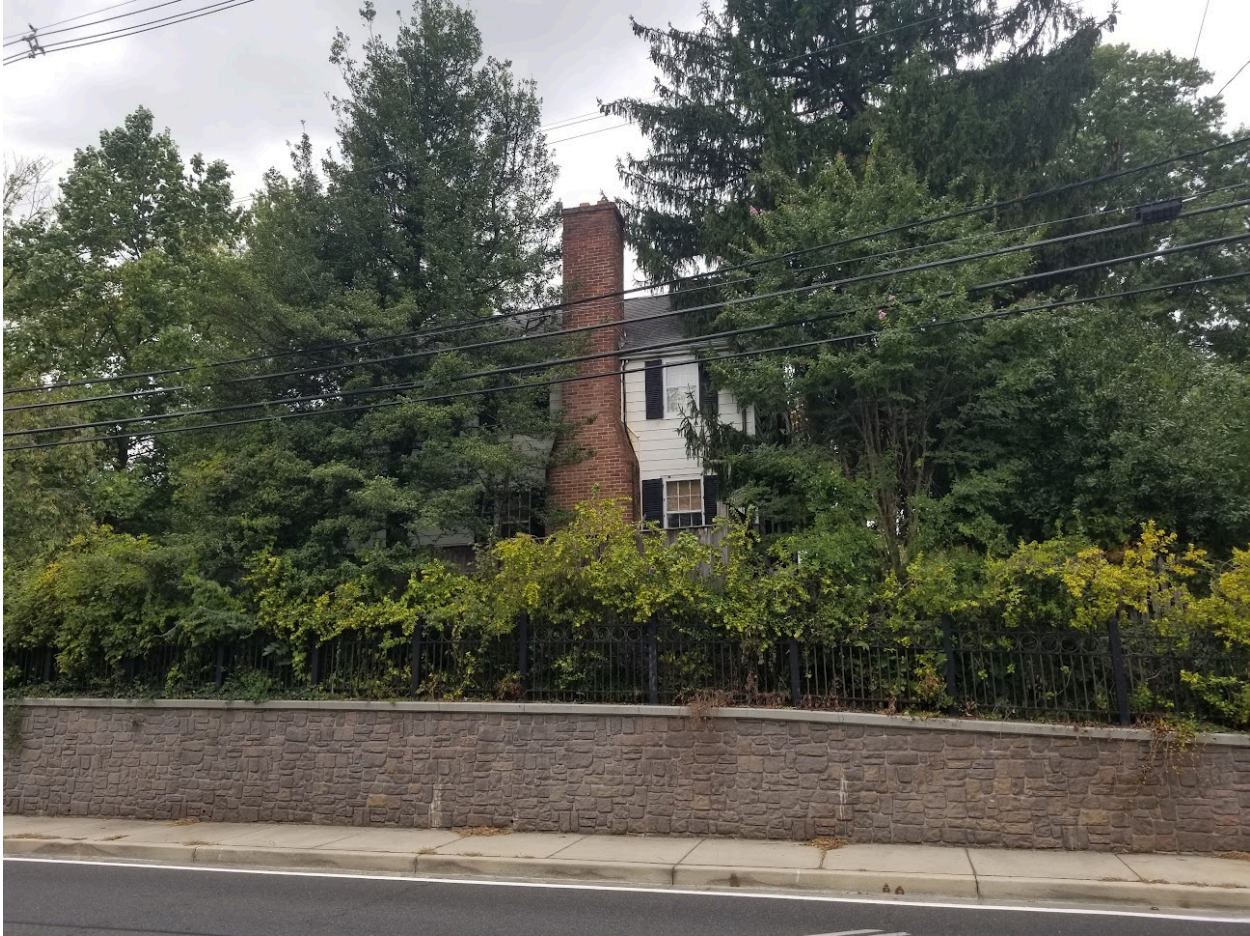
East side of the house from Connecticut Ave median
