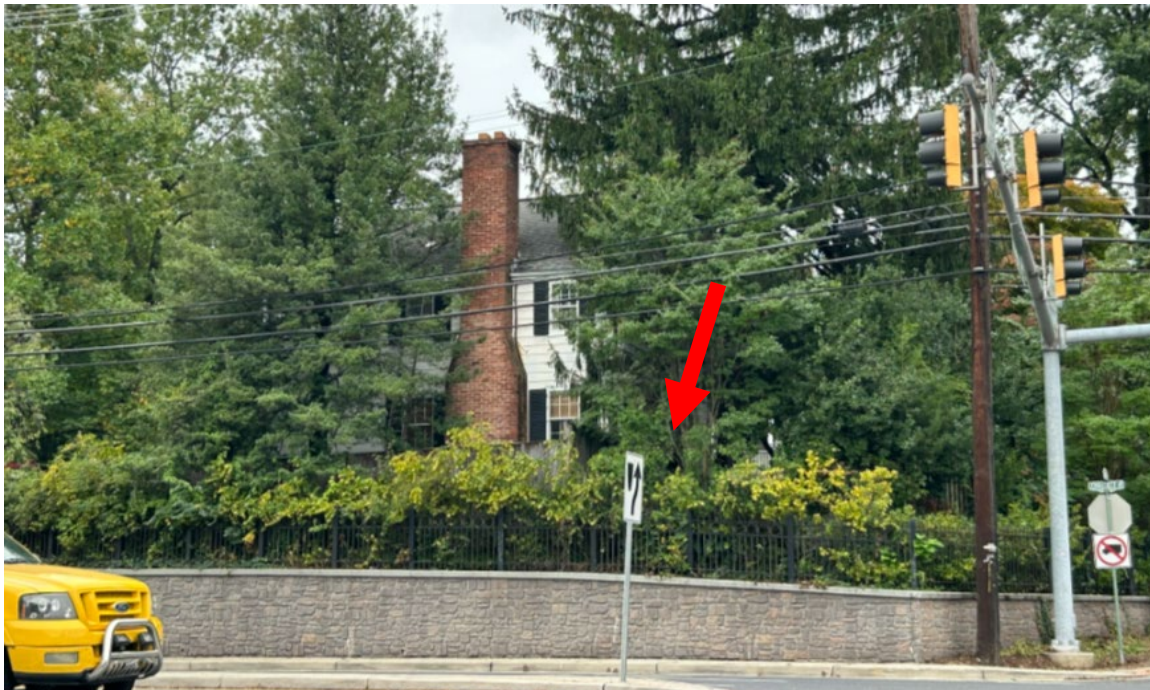
Figure 2: View west towards 3904 Washington Avenue from the intersection of Washington Street and Connecticut Avenue, September 2024 (Historic Preservation Office). A red arrow points to the approximate location of work.
