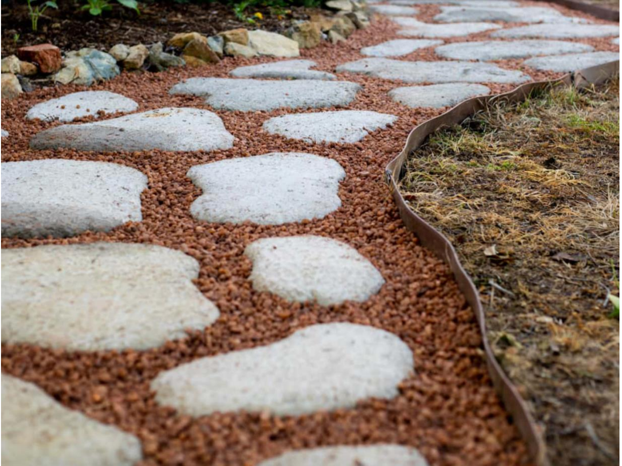
Concrete pavers for front walkway
