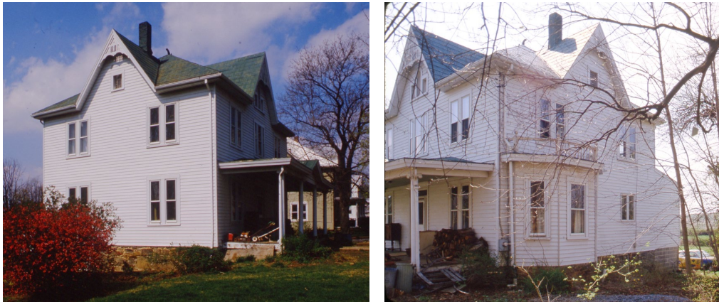
Figure 12: 19916 White Ground Road, features a main stone foundation and CMU foundation on rear addition.
