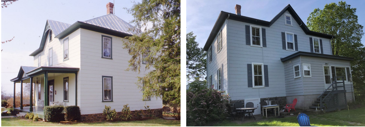
Figure 11: Front and side (left) and Rear (right) of the neighboring property at 1990 White Ground Road, showing the exposed stone foundation on the main block, and CMU foundation of the rear addition.
