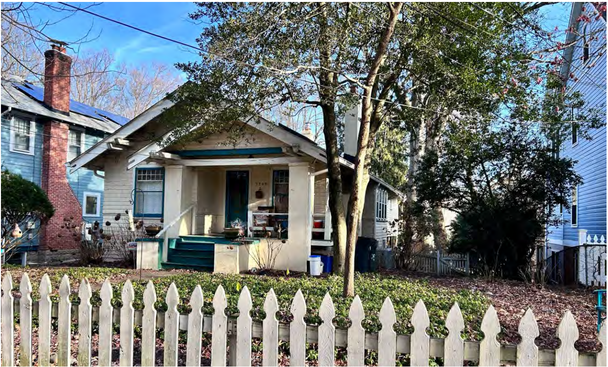
Figure 2: Front elevation of the subject property (Historic Preservation Office, December 2024).
