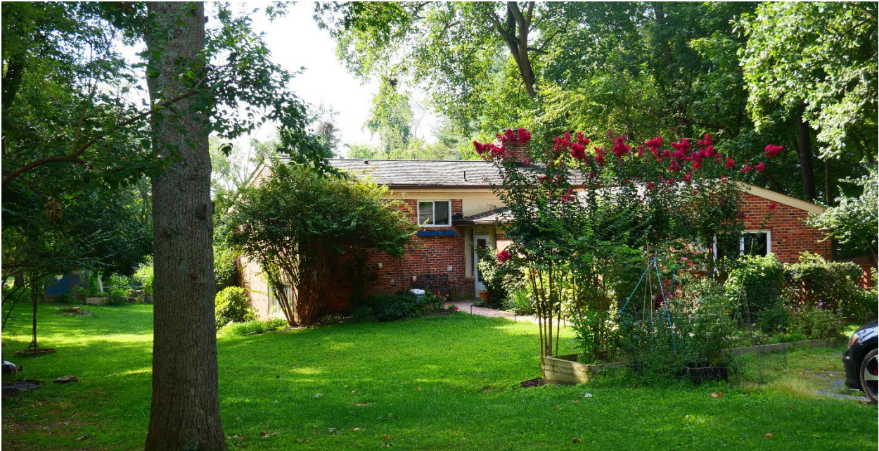
Figure 5: View of 12708 Running Brook Drive, 2024.
