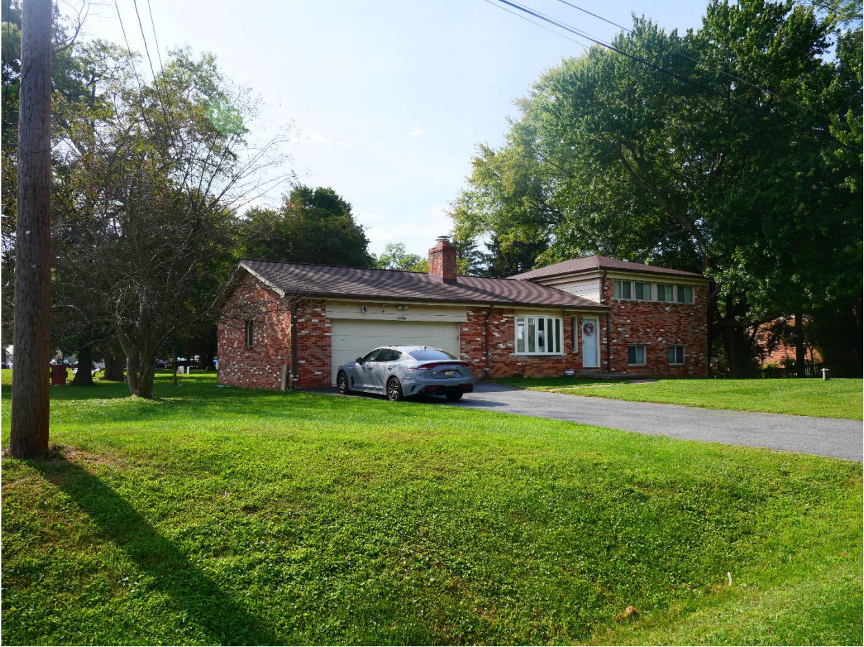
Figure 4: View of 12704 Running Brook Drive, 2024.
