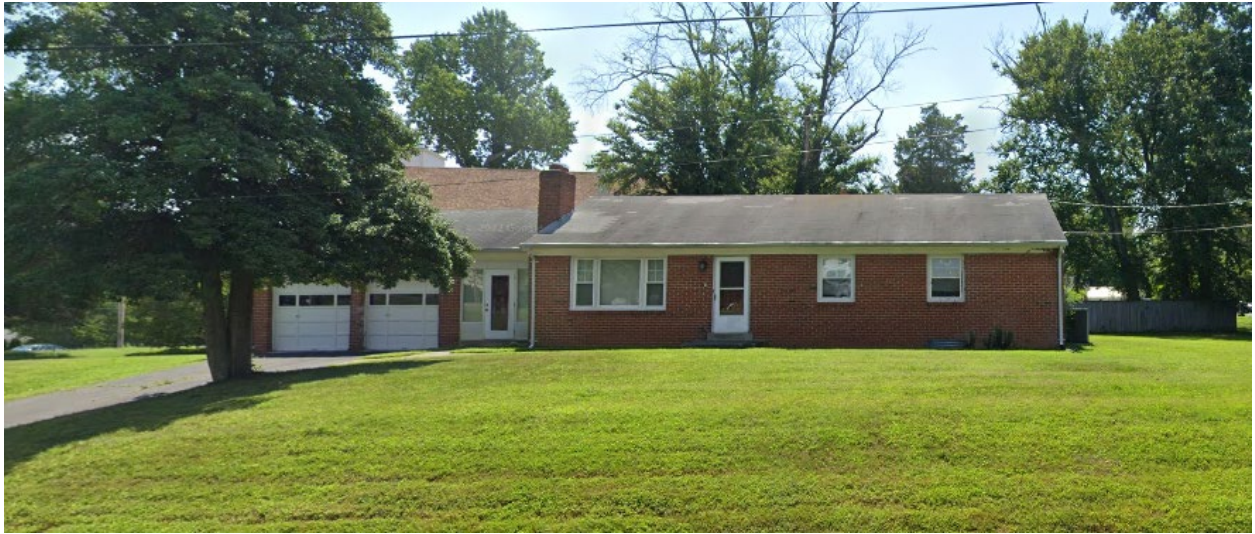
Figure 3: View of 12700 Running Brook Drive, 2024.
