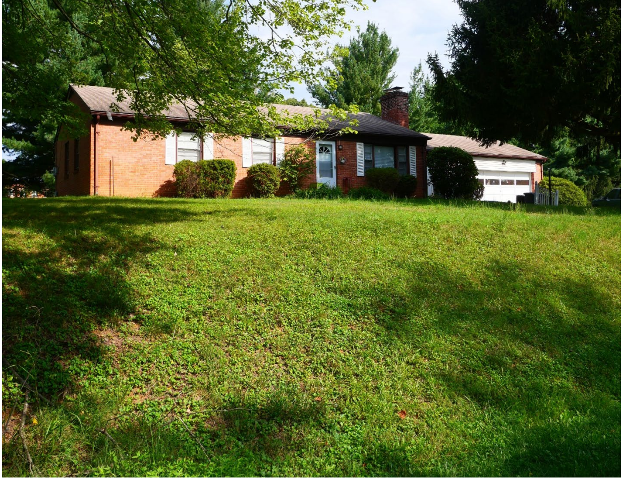
Figure 2: View of 12705 Running Brook Drive, 2024. The building appears to retain its original doors and windows.
