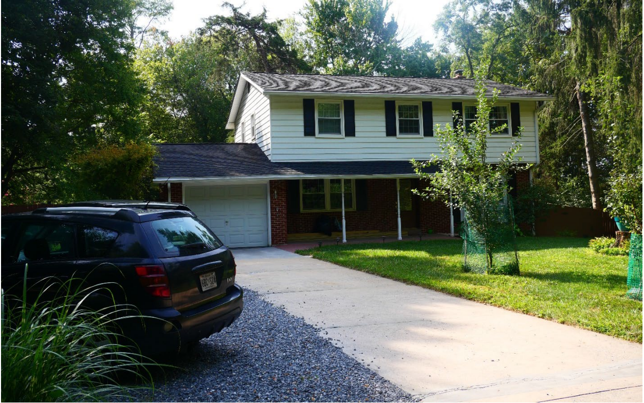
Figure 6: View of 12712 Running Brook Drive, 2024.
