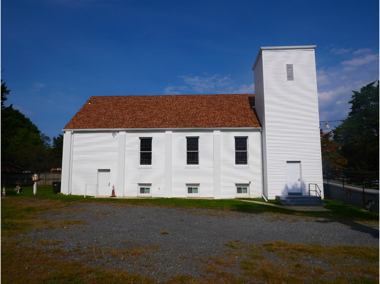
Figure 5: View of the side (south) elevation of Community of Faith United Methodist Church, 2024.
