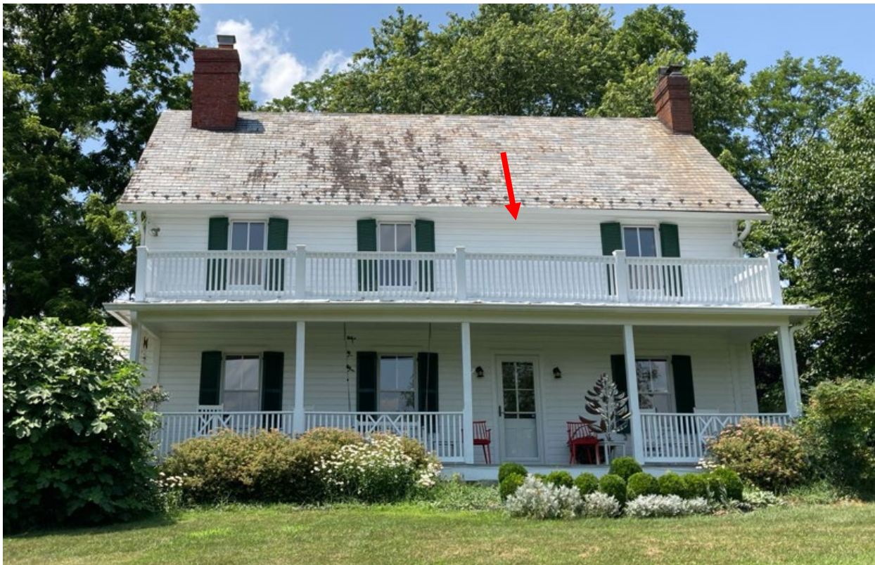
Figure 3: East elevation of the house. The red arrow points to the location of the proposed window.
