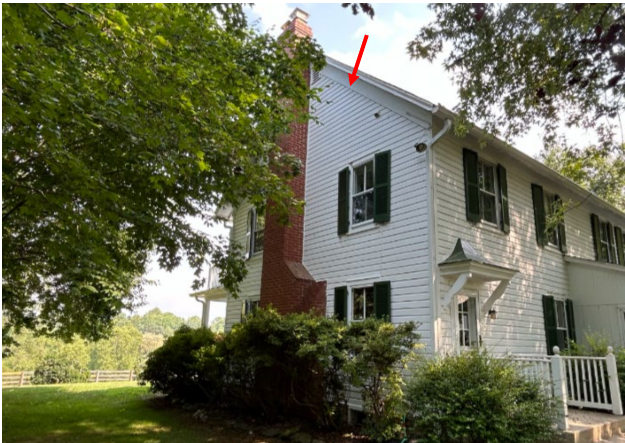
Figure 12: North elevation. The red arrow points to the location of the proposed casement window.
