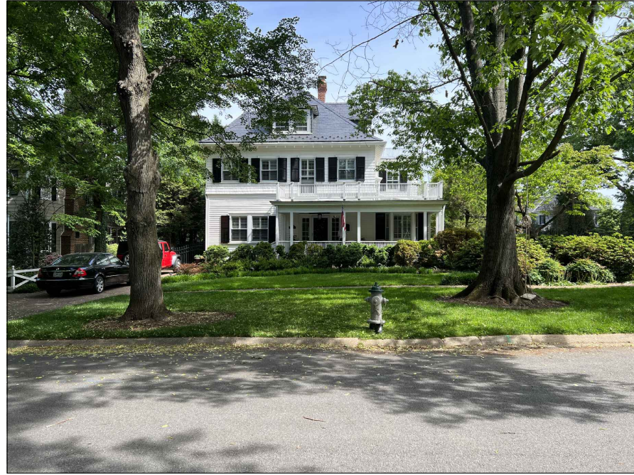
A1 A1|1 NTS EXISTING EXTERIOR VIEW - FRONT STREET VIEW
