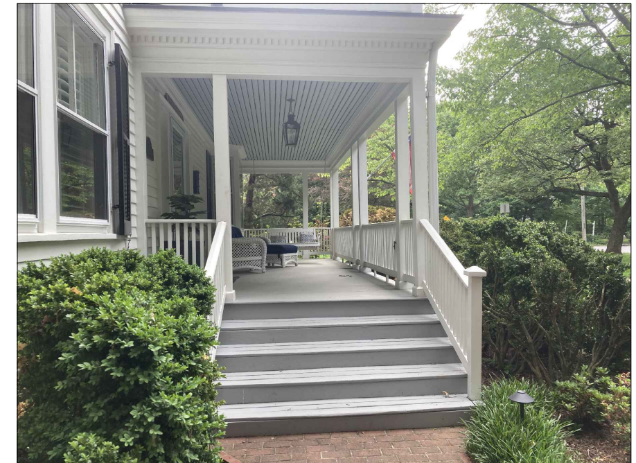
B3 A12 NTS EXISTING EXTERIOR VIEW - FRONT PORCH
