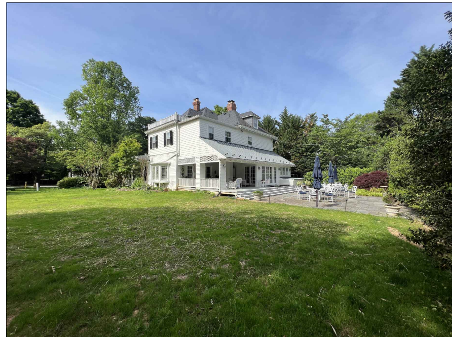
B2 A1|1 NTS EXISTING EXTERIOR VIEW - REAR SIDE LAWN
