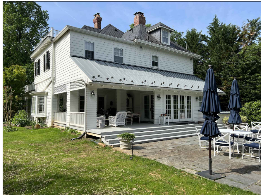
B1 A12 NTS EXISTING EXTERIOR VIEW - REAR
