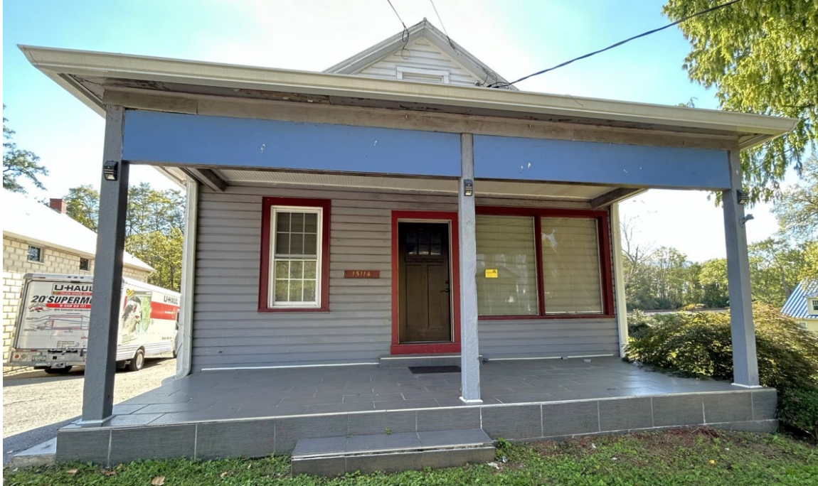
Figure 13: Front elevation, October 2024 (Historic Preservation Office).
