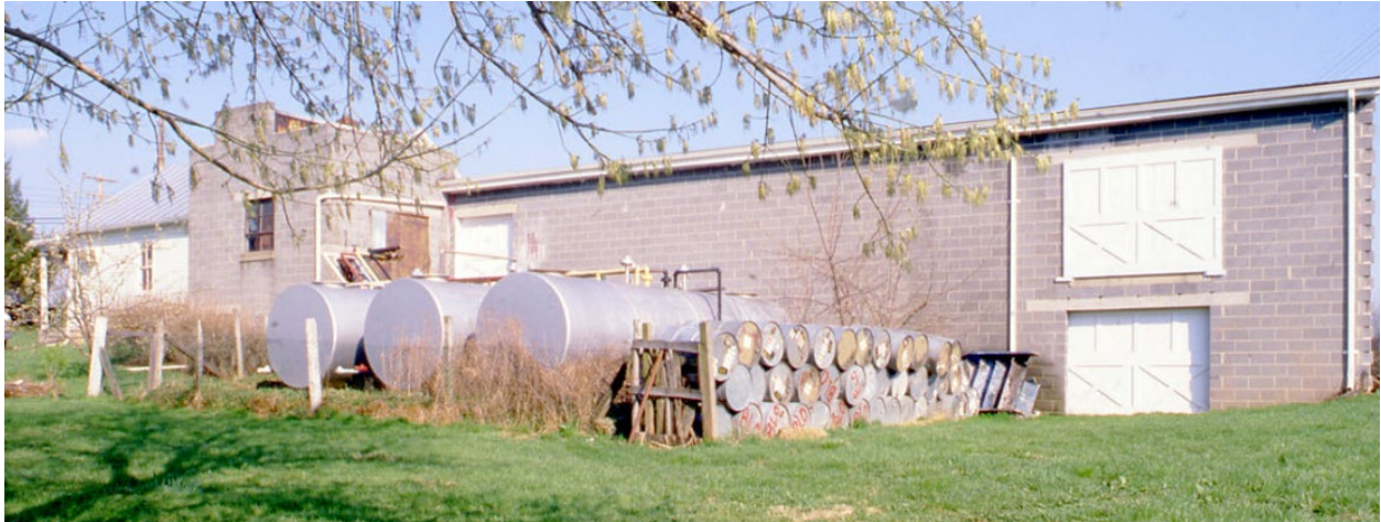
Figure 15: West side elevation of 15114 Barnesville Road, National Solvents Company, April 1986 (MCAtlas, Historic Preservation Office).
