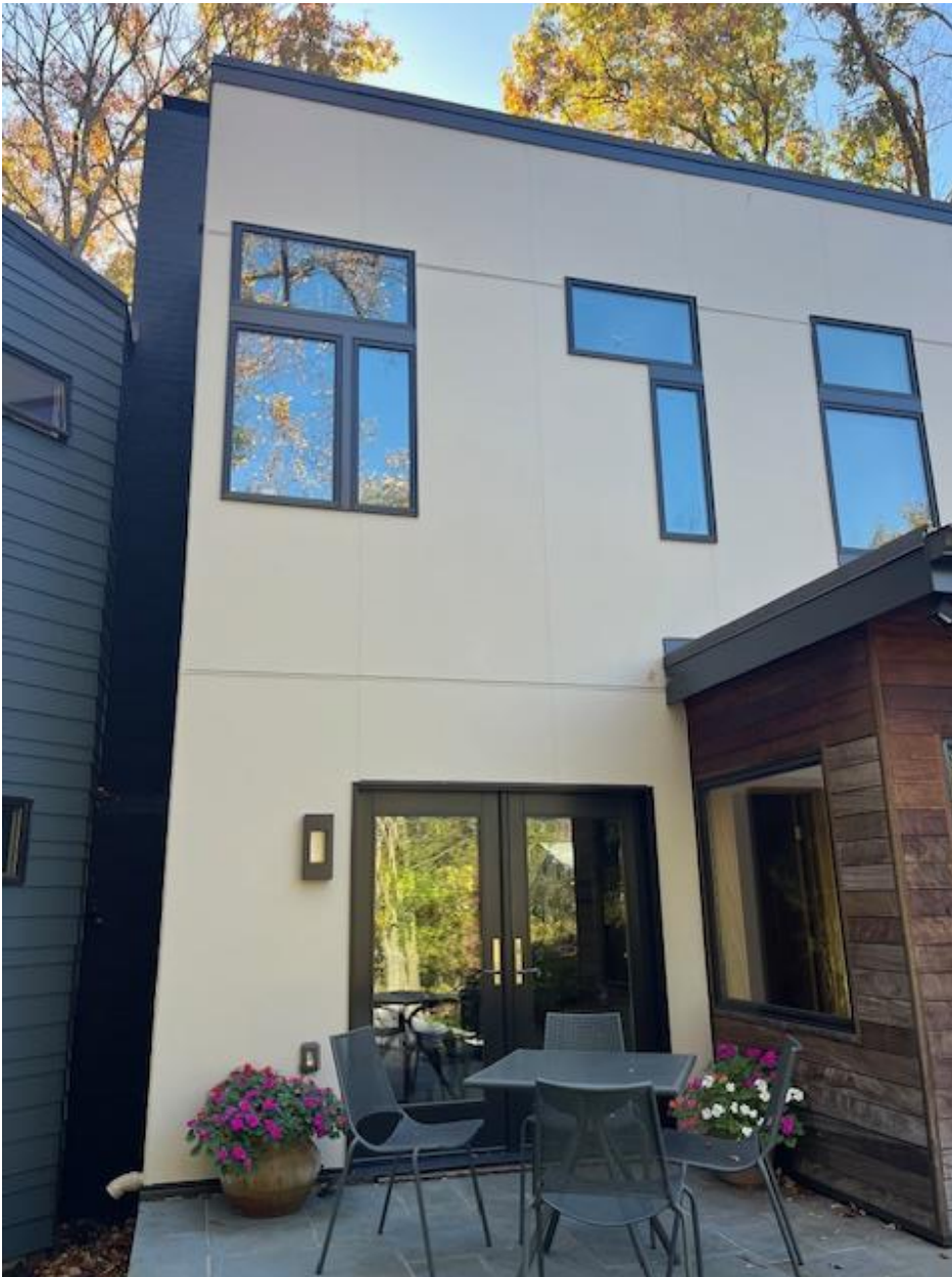
Caulked vertical joints between panels show a nearly seamless surface. Example from Garrett Park house.
