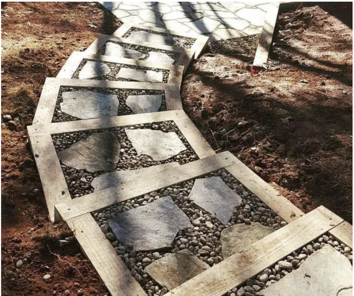
Steps for sloped side walkway
