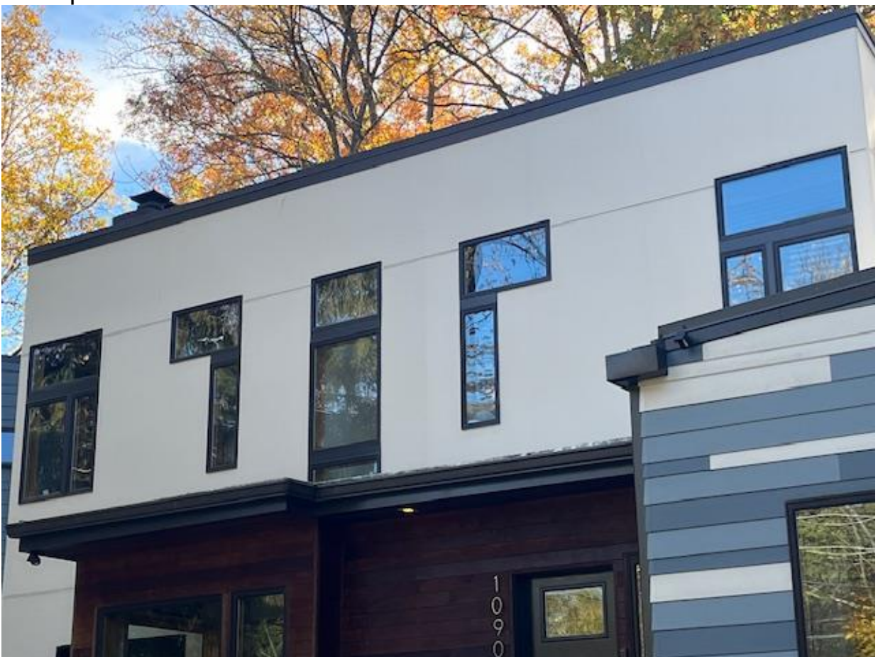
Caulked vertical joints between panels show a nearly seamless surface. Example from Garrett Park house.
