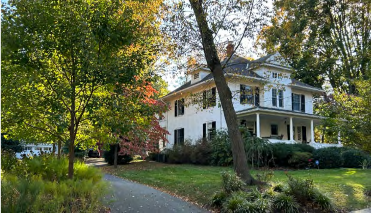
Figure 8: View of the east elevation from the end of the driveway.
