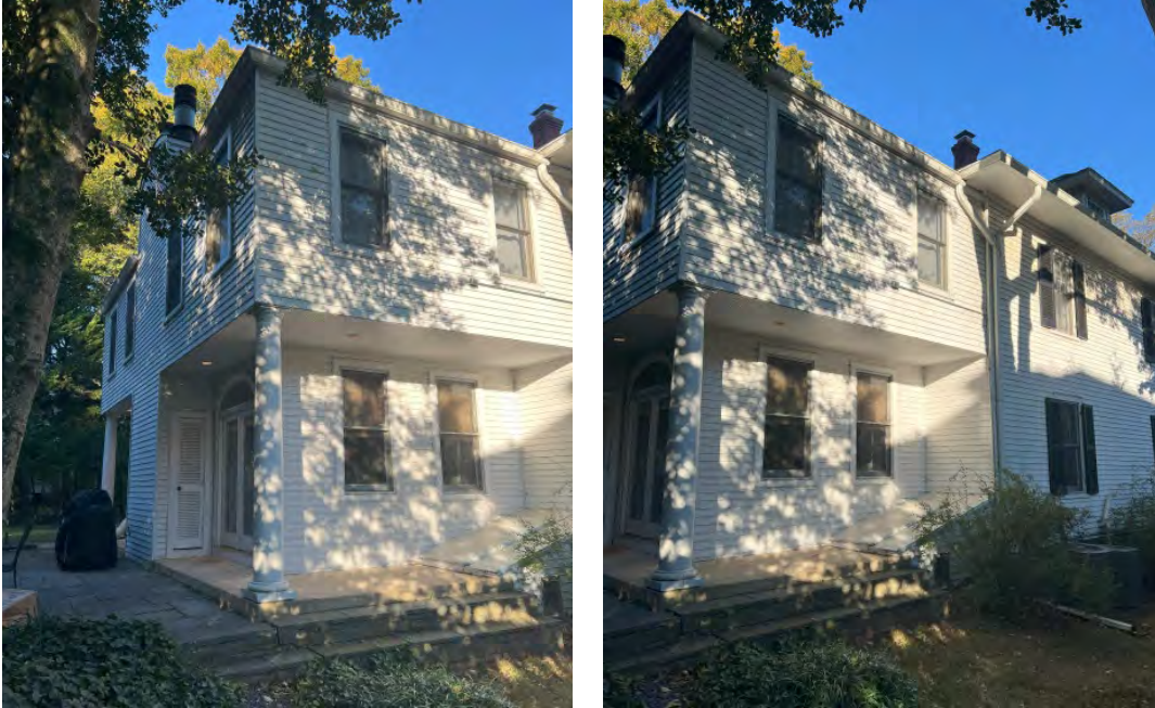
Figure 10: Existing east side rear addition and intersection with main block.
