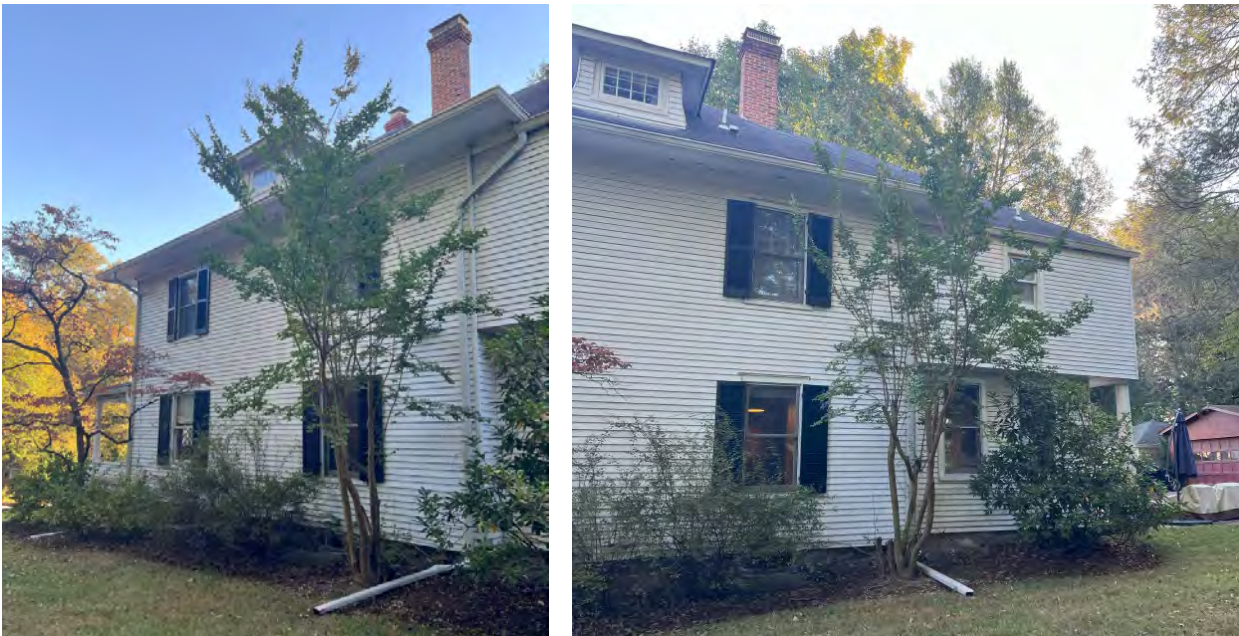
Figure 11: Photographs of the existing west side elevation.
