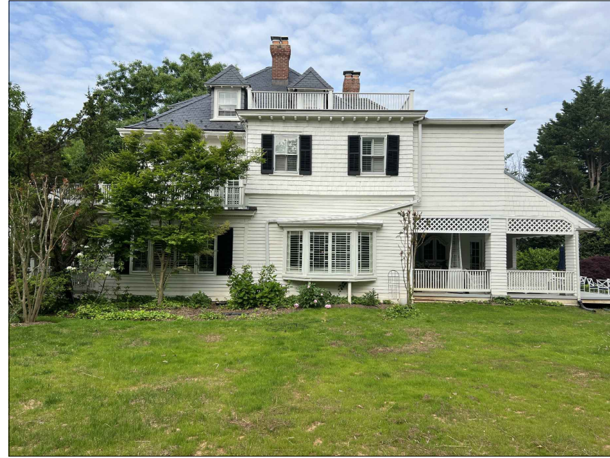
A2 A12 NTS EXISTING EXTERIOR VIEW - WEST
