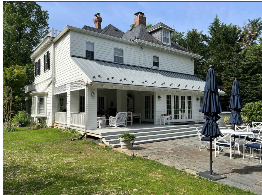
B1 A12 NTS EXISTING EXTERIOR VIEW - REAR
