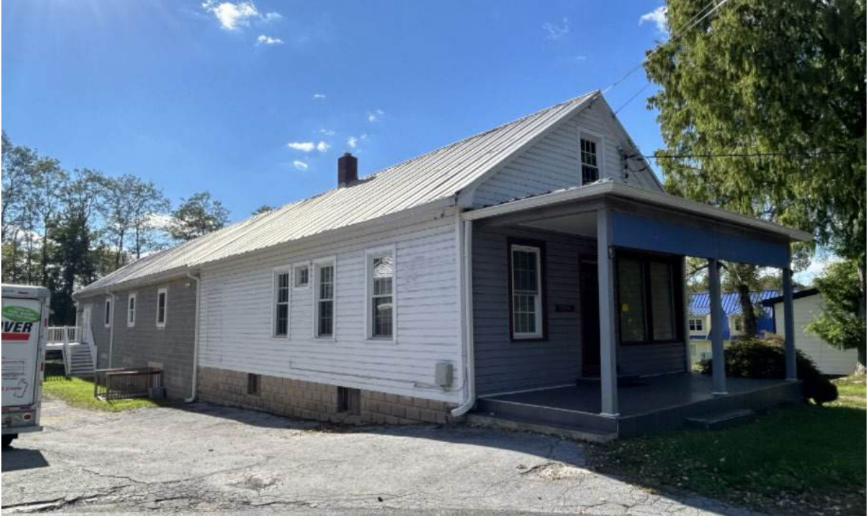
Figure 4: 15114 Barnesville Road, front (north) and east side elevations, October 2024 (Historic Preservation Office).
