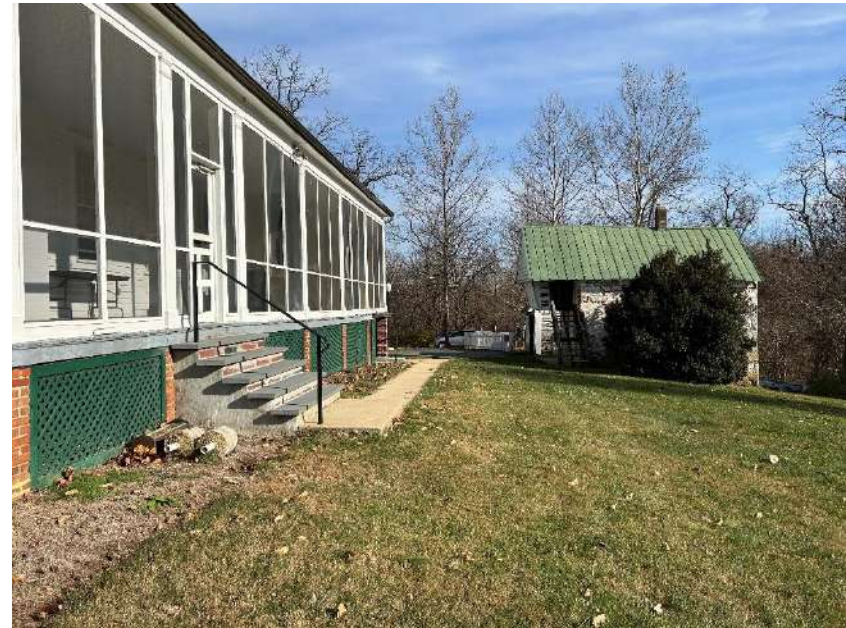
View East towards Dairy and Parking
