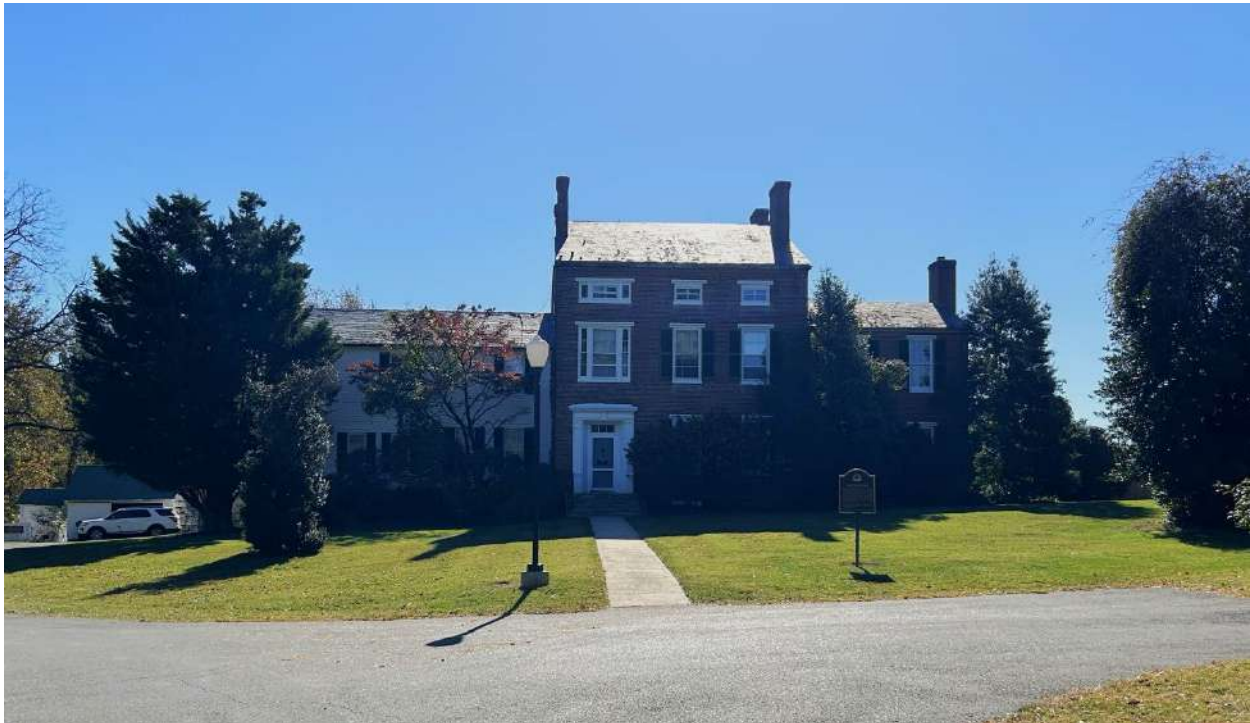
Figure 1: Front (north) elevation of Needwood Mansion.
