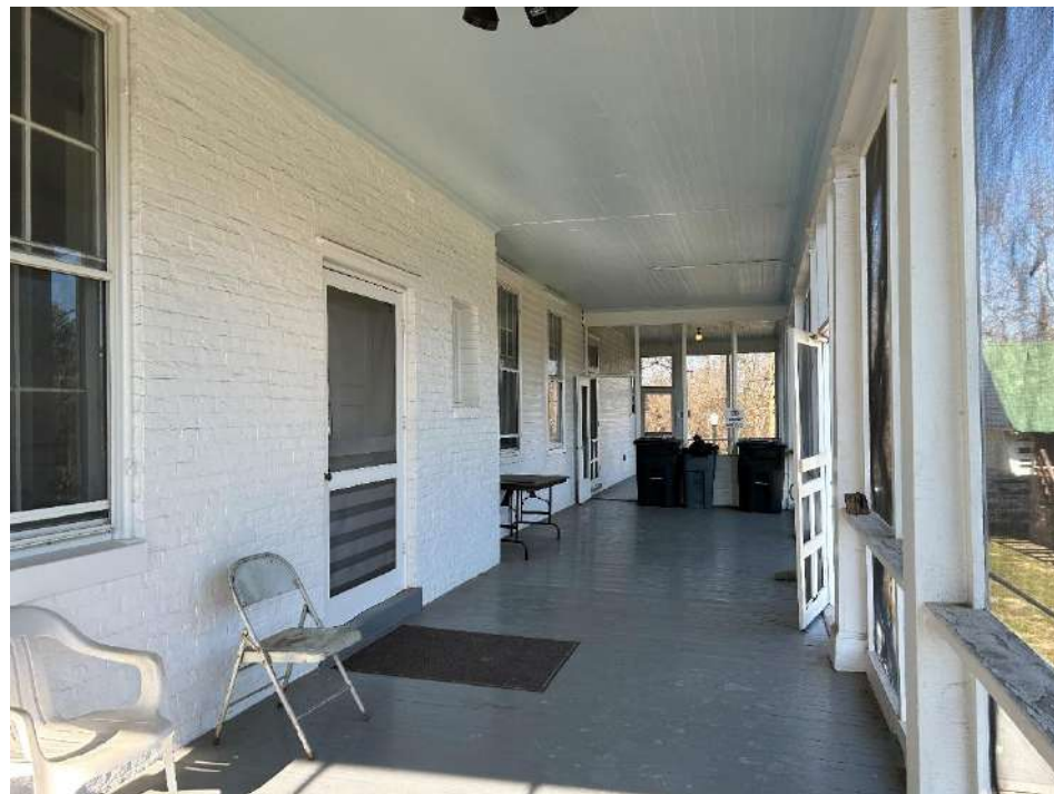
Main Porch Area at Center Block, Main House Entry on Left
