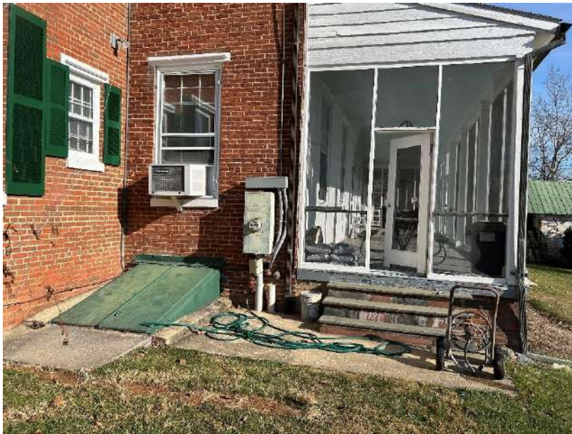
West Porch Stair
