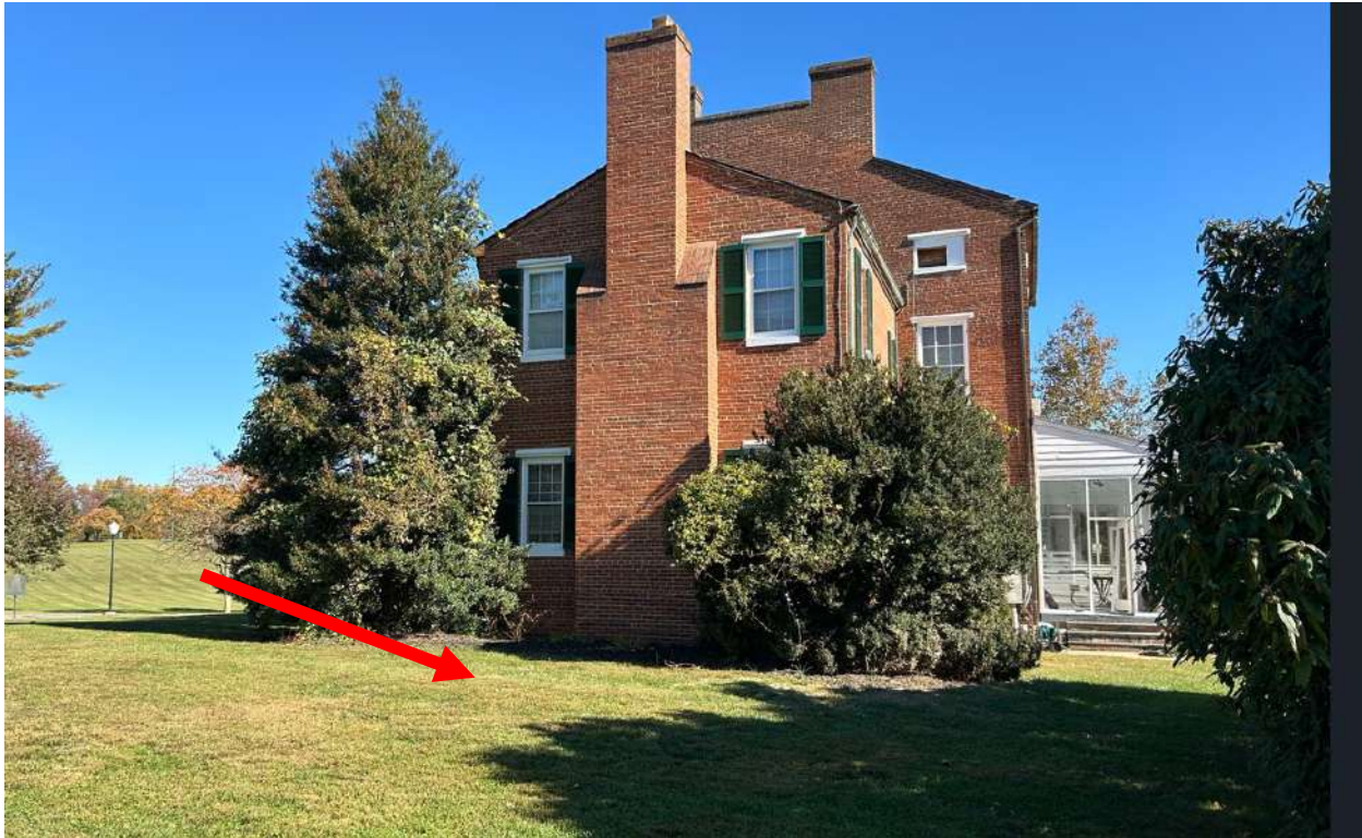
Figure 10: View of the proposed equipment enclosure location at the west end of the building.
