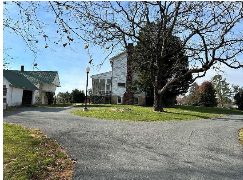
East Elevation (from Parking Lot)
