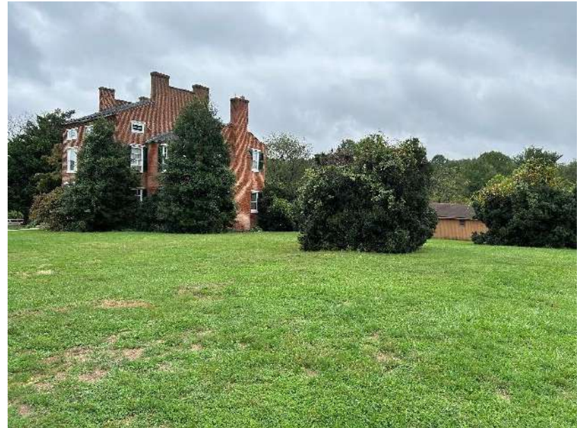
North Lawn, Looking to West Elevation
