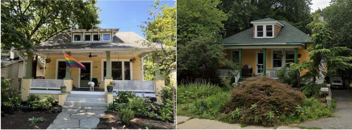
Figure 2: 7100 Sycamore (left) and 7108 Sycamore (right), Craftsman houses with wood railings and balusters.
