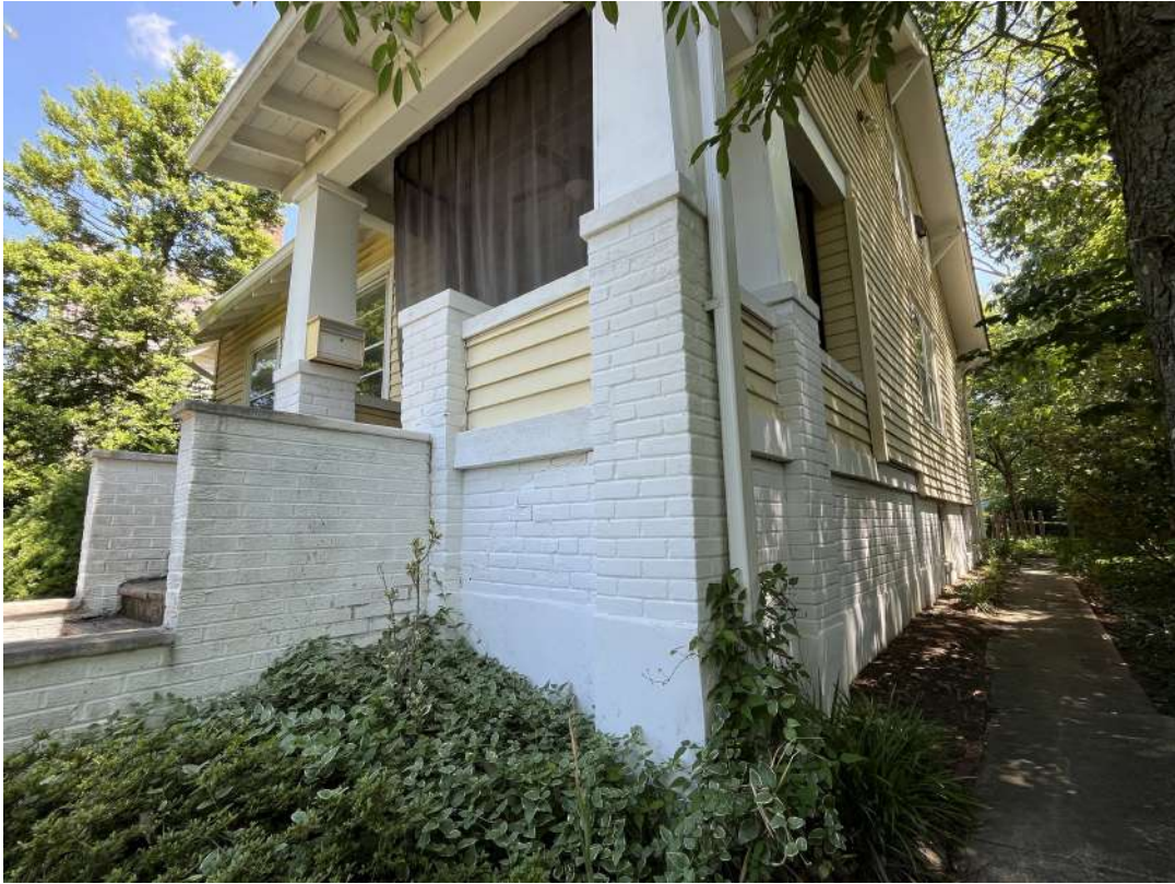
Detail: 7017 SYCAMORE AVE. FRONT PORCH CLOSE-UP
