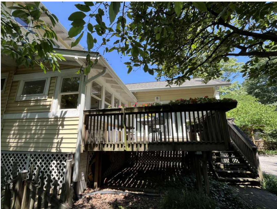
Detail: 7017 SYCAMORE AVE. SOUTH-REAR DECK CLOSE-UP
