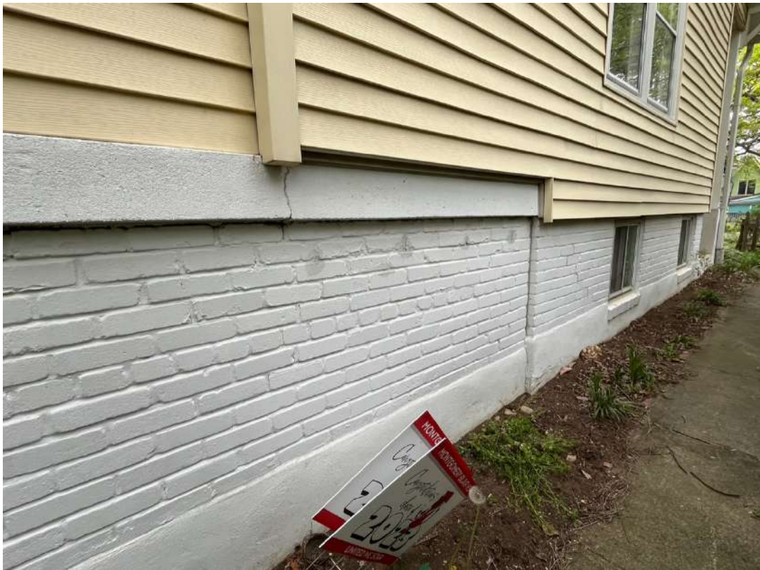
Detail: 7017 SYCAMORE AVE. FOUNDATION
