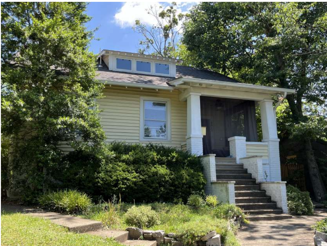
Detail: 7017 SYCAMORE AVE. FRONT PORCH
