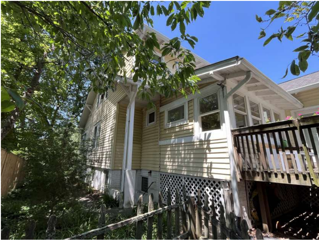
Detail: 7017 SYCAMORE AVE. SOUTH-REAR DECK
