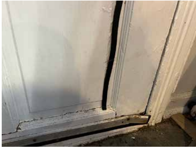
Poor fit with frame, many cracks in door, stickers on window
