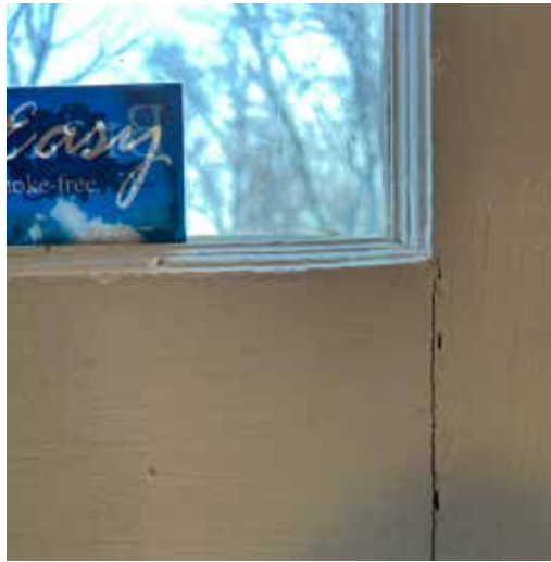
Poor fit with frame, many cracks in door, stickers on window
