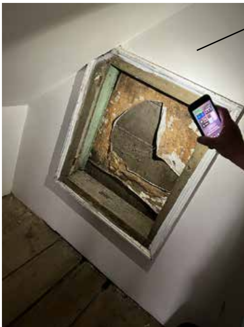
Left window frame (covered by aluminum siding on outside of house)
