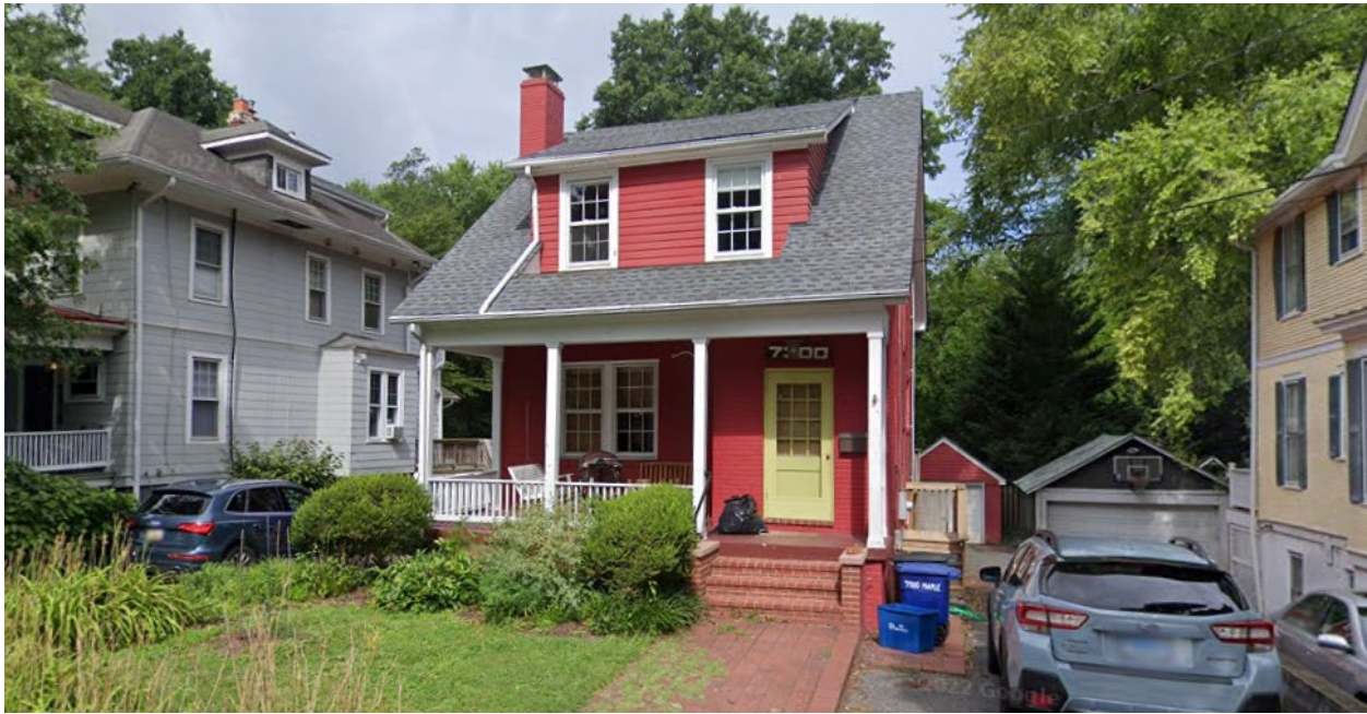
Figure 2: The front (southeast) elevation of 7300 Maple Avenue.
