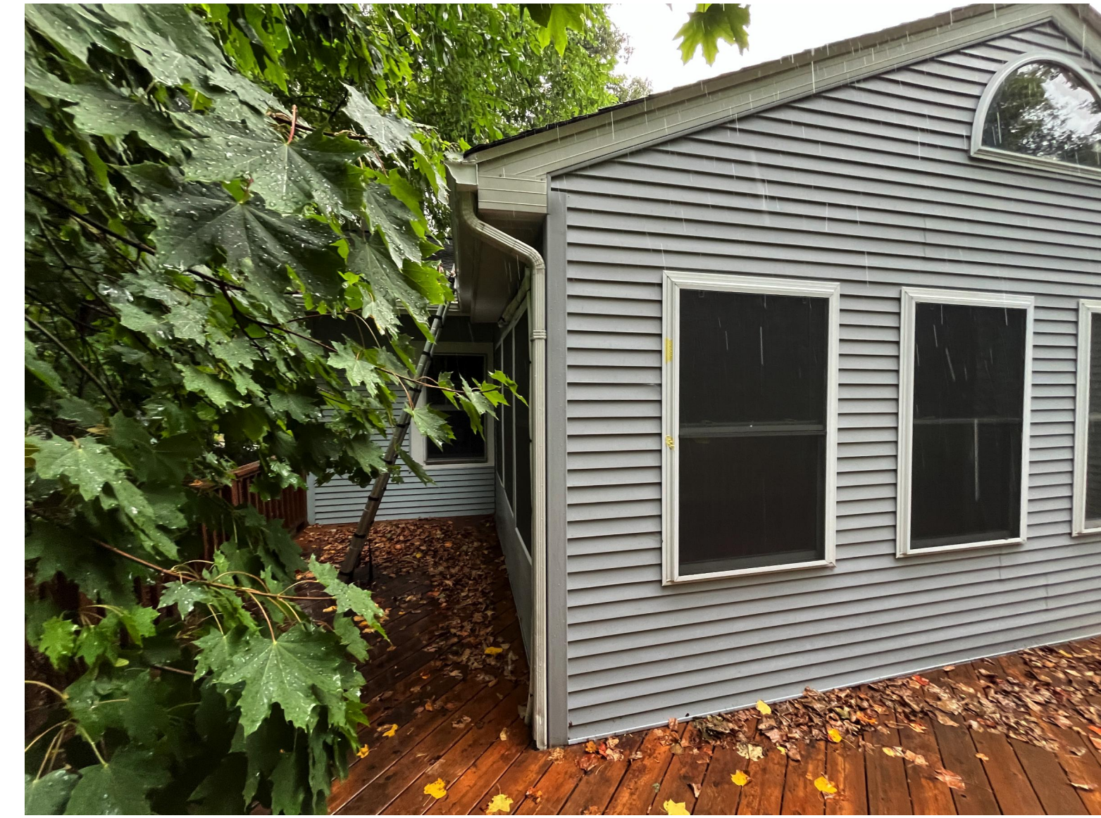
REAR (WEST) ELEVATION CONTINUED
