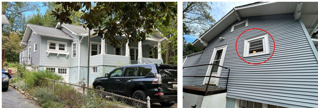
Figure 11: Location of the window to be removed on the south elevation of the historic building.
