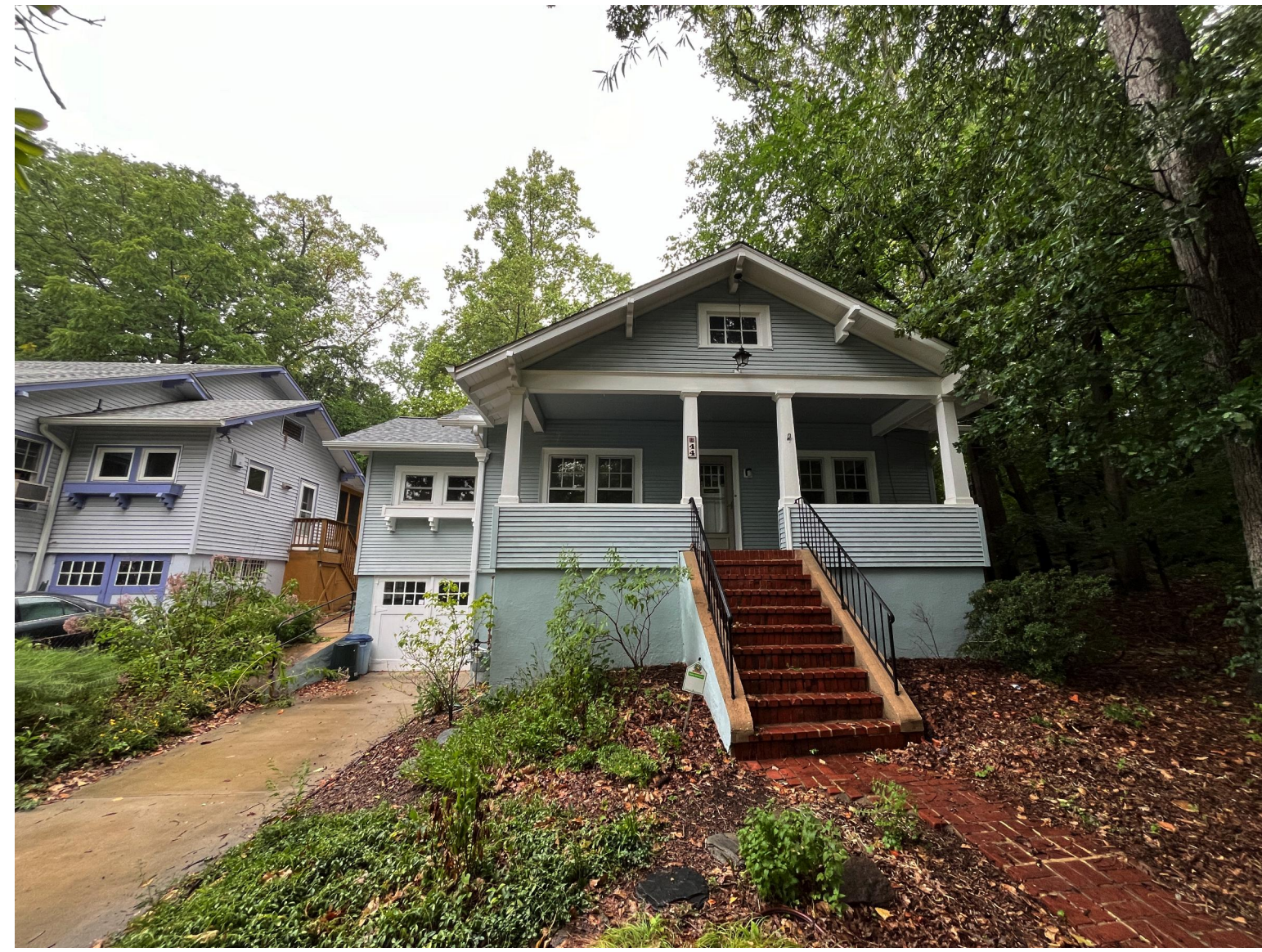
FRONT ENTRY AND EAST ELEVATION ALONG COLUMBIA AVENUE
