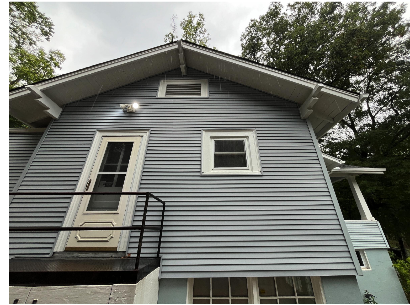
SIDE (SOUTH) ELEVATION LOOKING AT DOOR TO EXISTING KITCHEN
