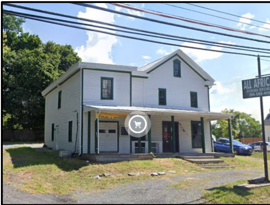
Figure 9: The Contributing Resource at 23341 Frederick Road is an examples of a two-story commercial building in the Clarksburg Historic District. Source: Google
